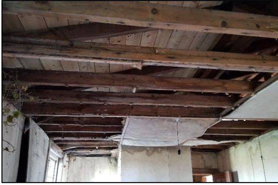
Figure 6: Internal view – rooms open to roof structure.
