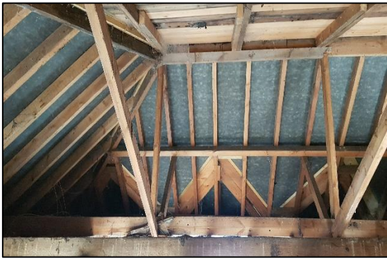
Figure 8: View of roof structure – felt lining.
