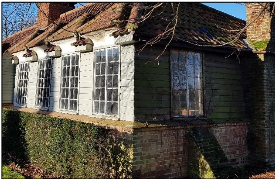
Figure 3: Painted and untreated weatherboarding – tightly sealed.
