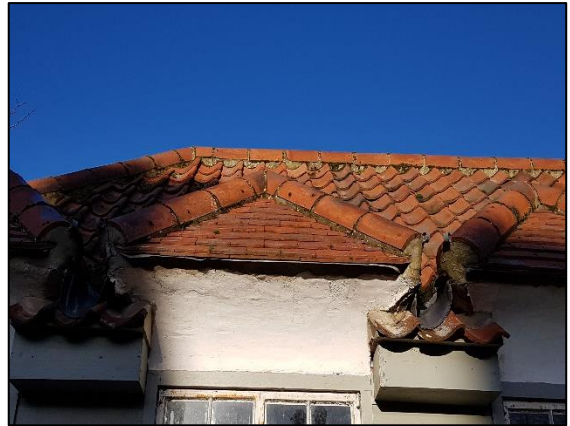
Figure 4: Tiles above windows
