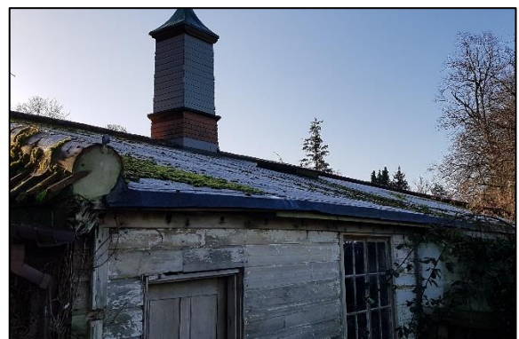
Figure 2: Rear view of lined roof.
