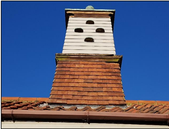
Figure 3: Hanging tiles on turret.
