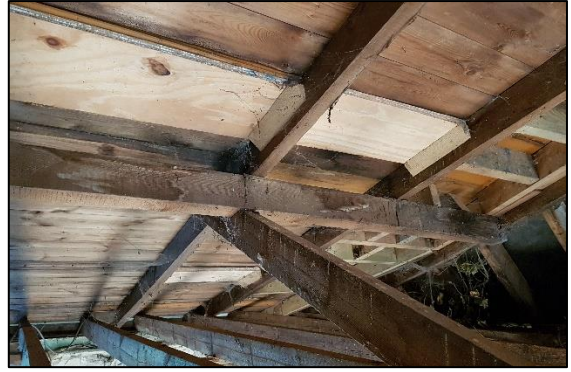
Figure 7: View of roof structure – wooden lining.
