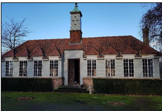
Figure 1: Dovecote Cottage – southern aspect (front).
