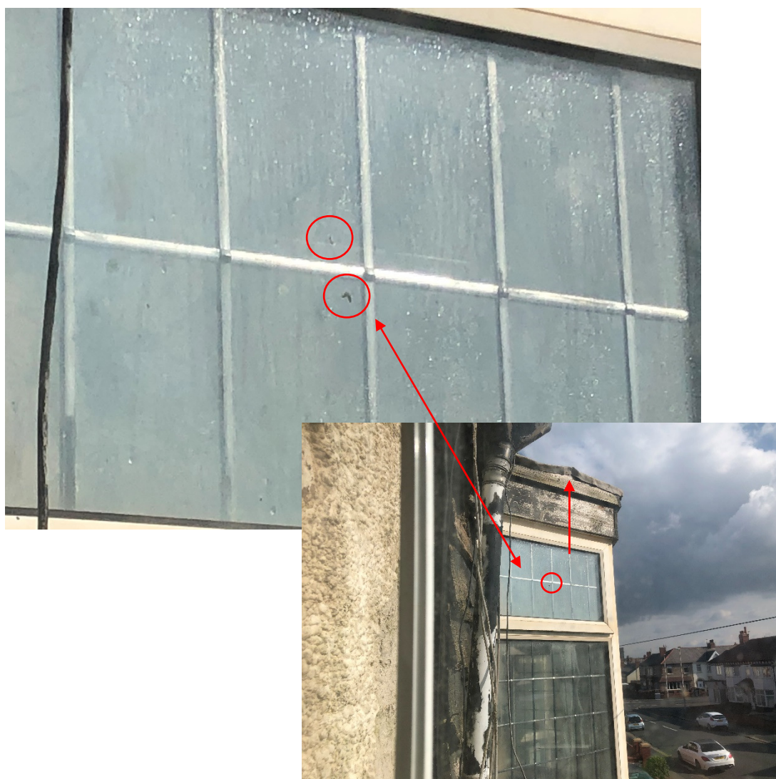
Photograph No.9: Potential bat droppings (x2) attached to second floor window of No.8 on the southern façade, as viewed from the upstairs of No.6. Lead flashing has lifted above location of the droppings and is considered to offer suitable ingress for crevice dwelling bat species.
