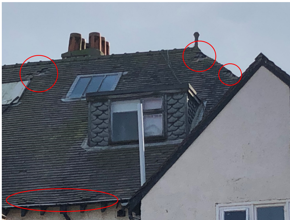
Photograph No.3: Rear of No.6, looking south.
