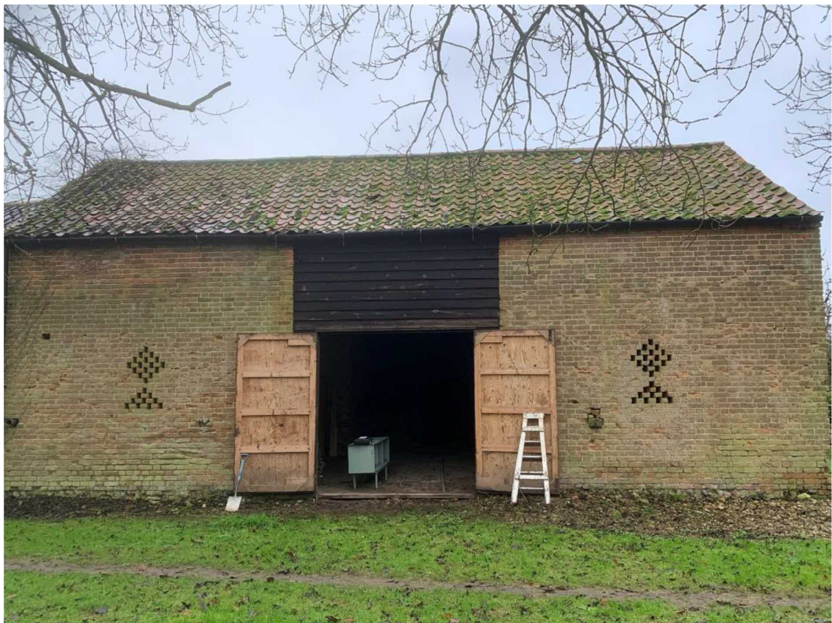
North Elevation of Building
