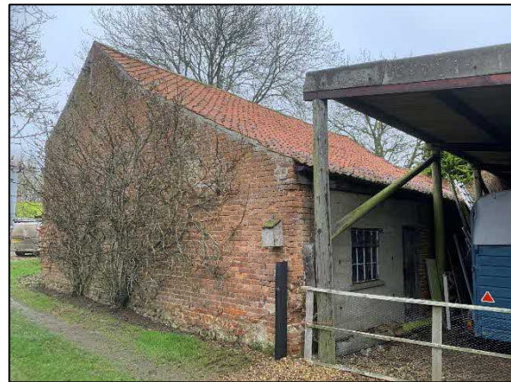
Figure 2. Southern and western aspects
