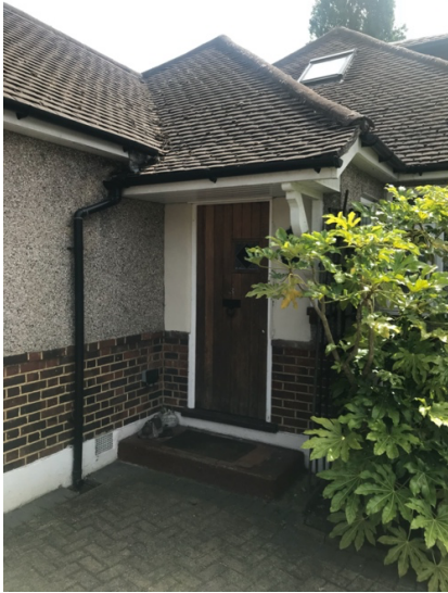
Figure 1: Stepped up entrance door
