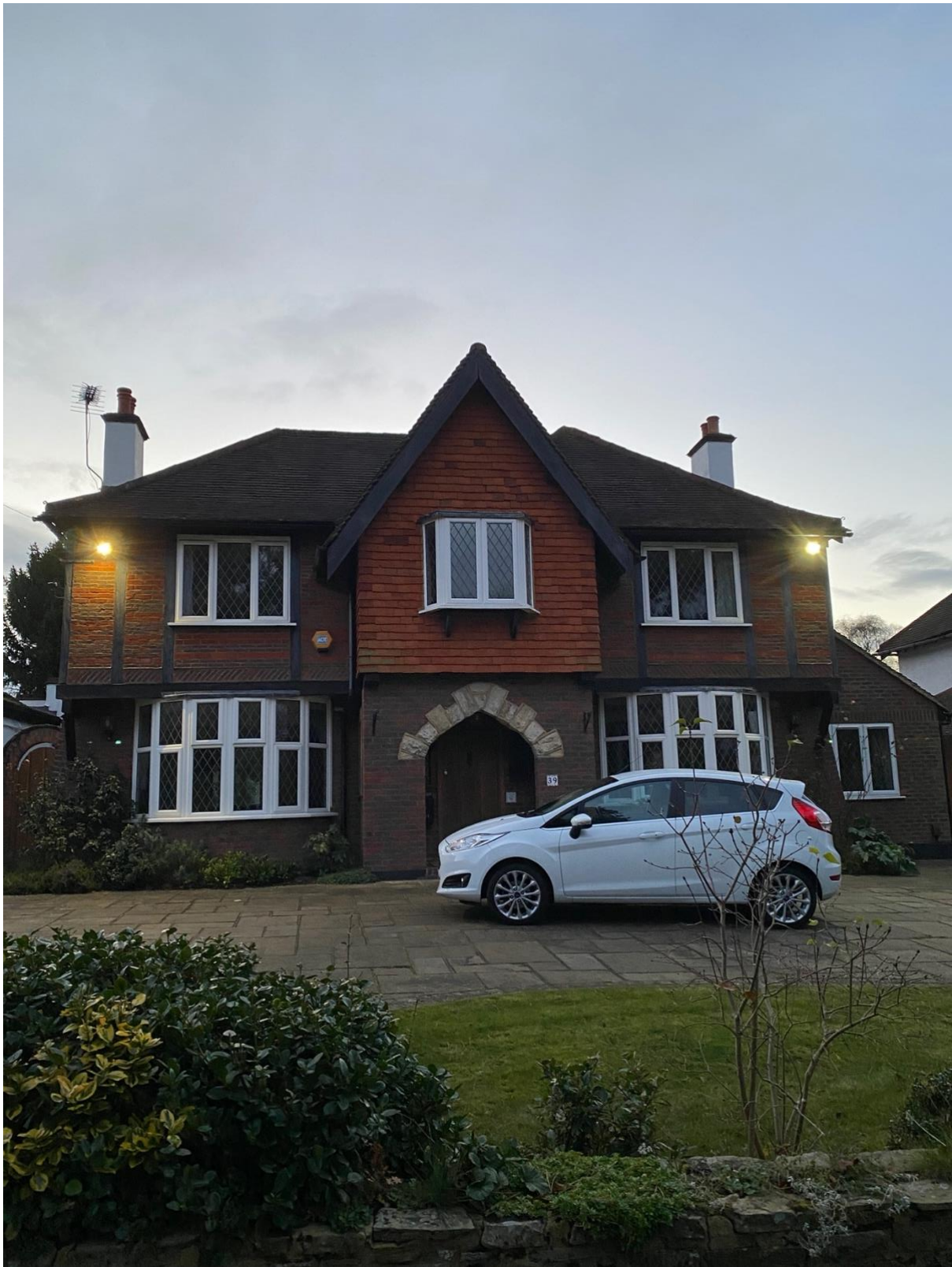
HB211023 – SITE PHOTOS (taken DEC 2021)
