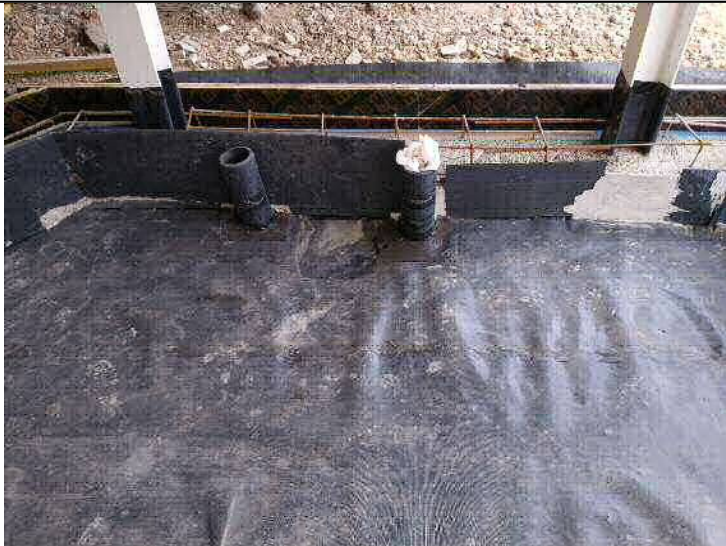
Photograph 19 – Membrane and service entry, Slab D.
