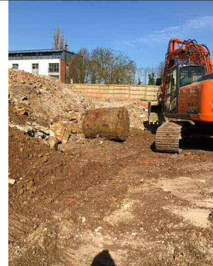
Photograph 4 – Adston Construction photo of tank T4.
