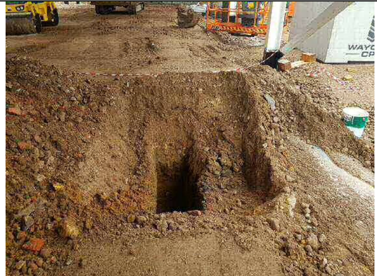
Photograph 8 – A view of part of TP402.
