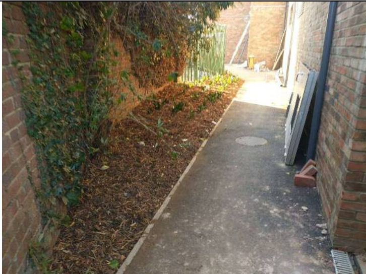
Photograph 7 – A general view of Area 4.
