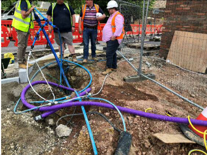
Photograph 1 – Lidl photograph of installed Protecta-Line Barrier Pipe
