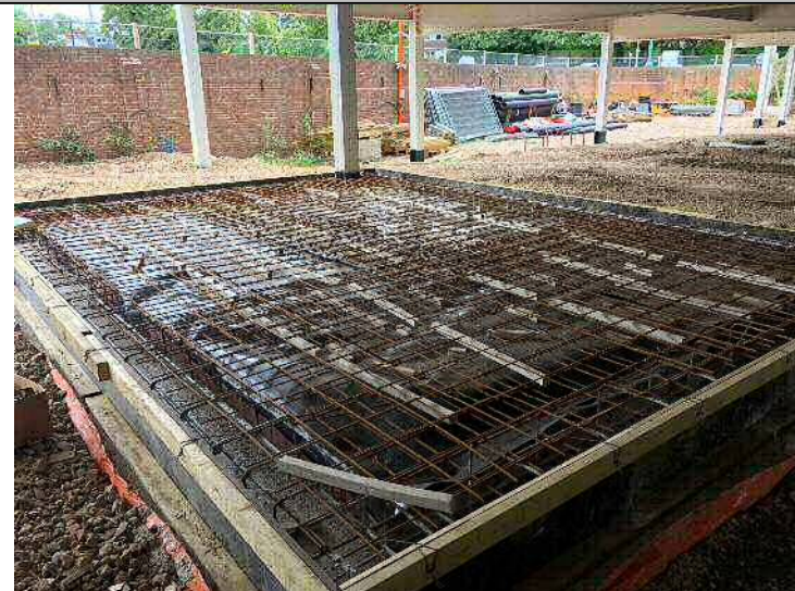
Photograph 16 – A view of Slab C (steel work installed prior to arrival)
