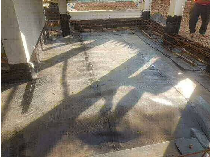
Photograph 21 – A view of the membrane installed in Slab H.
