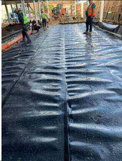
Photograph 13 – A view of the first section of Slab A
