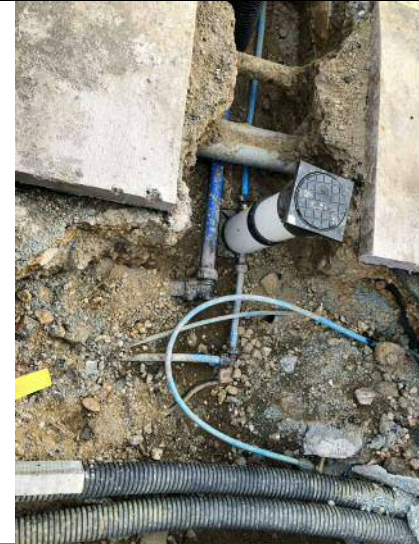
Photograph 2 – Lidl photograph of installed Protecta-Line Barrier Pipe
