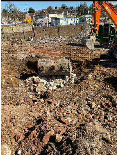
Photograph 3 – Adston Construction photo of tank T1-T3.
