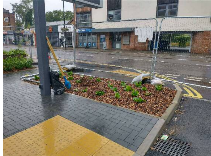
Photograph 2 – Hand pit location and general view of Area 1
