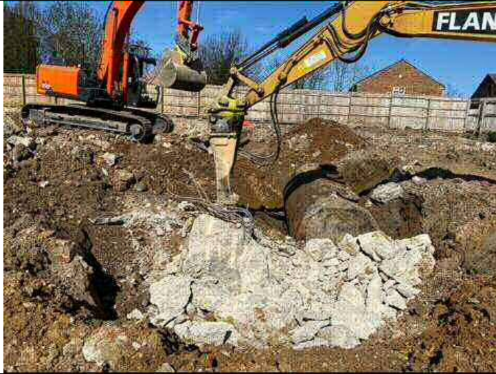
Photograph 1 – Adston Construction photo of breaking out around tank T1-T3.
