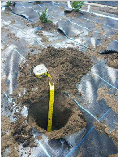
Photograph 11 – Hand pit in Area 5.
