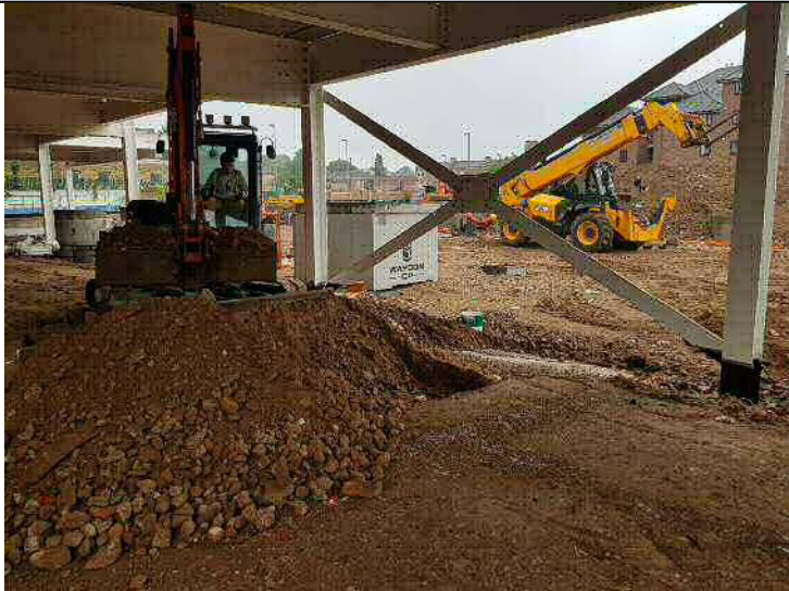
Photograph 7 – A view of TP402 location.
