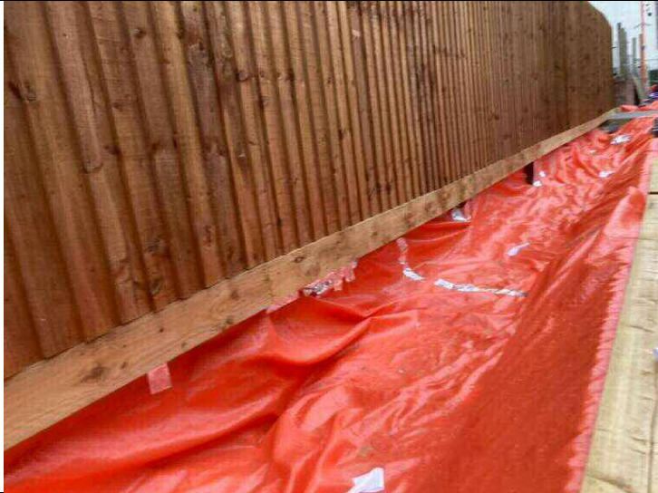
Photograph 1 – Adston construction photo of FasTrack Orange Geotextile installation
