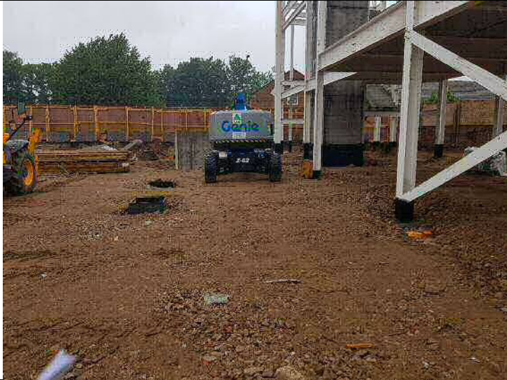
Photograph 5 – A view of TP401 location.
