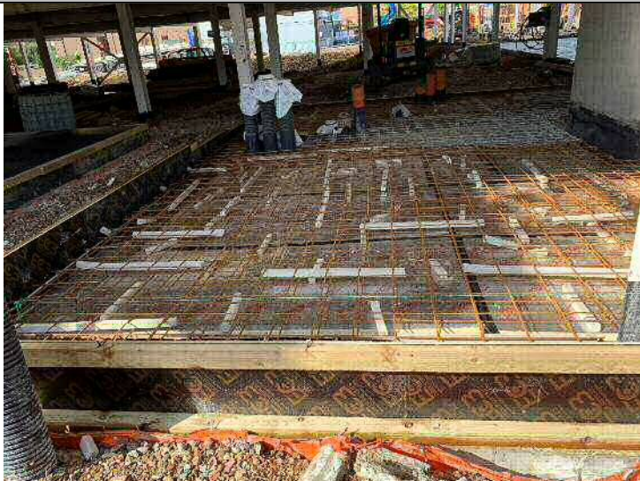
Photograph 15 – A view of Slab B (steel work installed prior to arrival)
