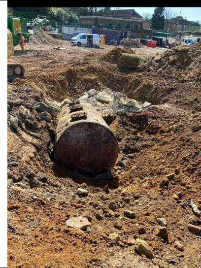
Photograph 2 – Adston Construction photo of tanks T1-T3 (foreground) and T4 (background).
