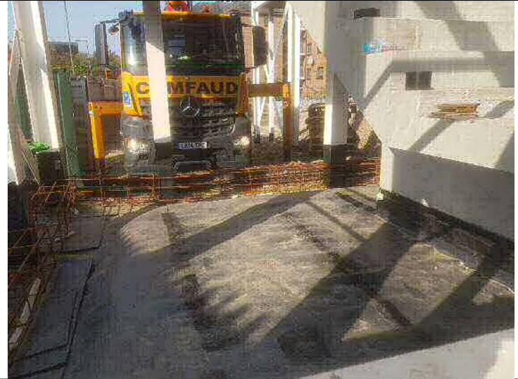
Photograph 22 – A view of the membrane installed in Slab H.
