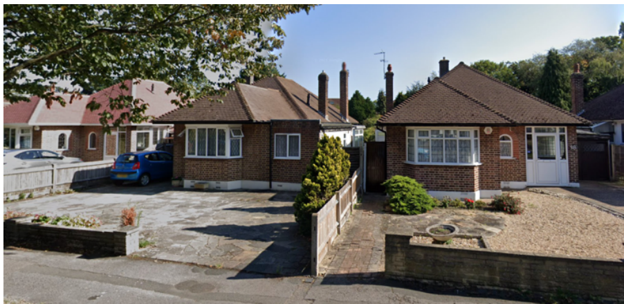
Figure 6: Flat roofed side extension also with front-facing parapet at No.40 Salisbury Rd
