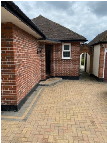
Figure 1: View towards the main entrance
