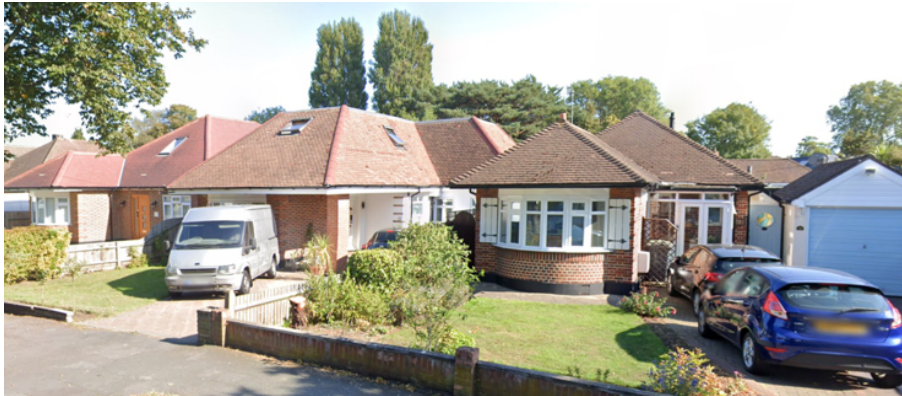
Figure 5: Crown roof to remodelled No.22 Salisbury Rd (left centre)
