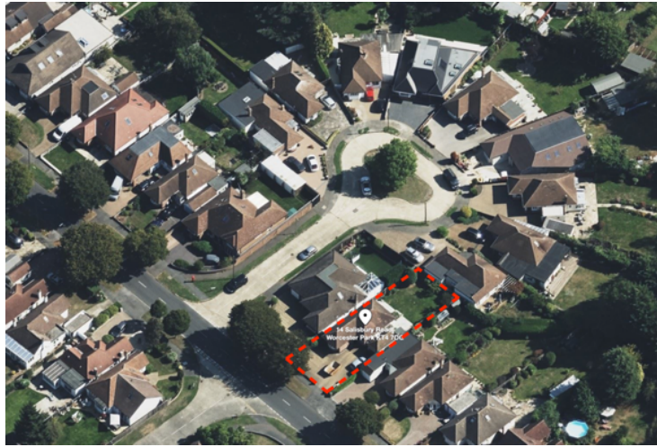
Figure 8: Various roof forms to extended properties on Salisbury Rd and Plantagenet Cl. ( Bing Maps )
