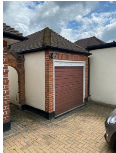
Figure 2: Detached storage Garage
