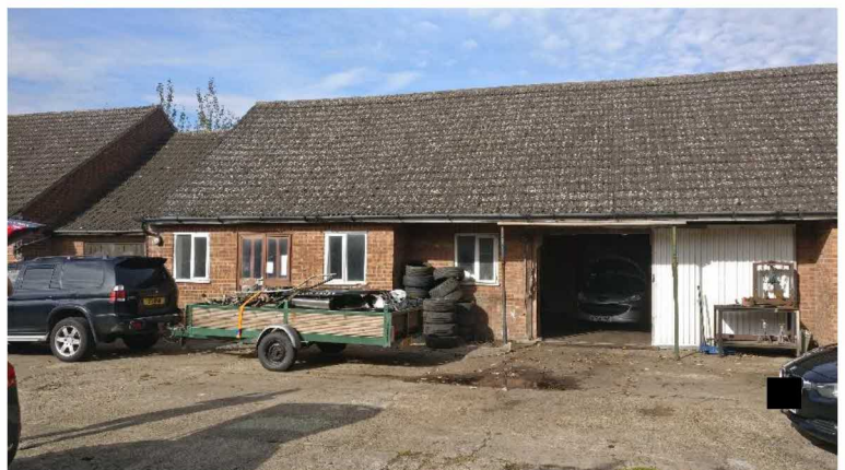
53 Crossdale Street with store adjoining to the south (to be demolished)
