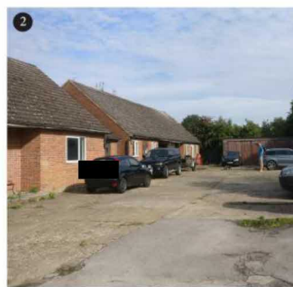
View of AG tool hire from site access
