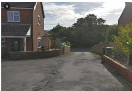
View of access towards Norwich Road A149
