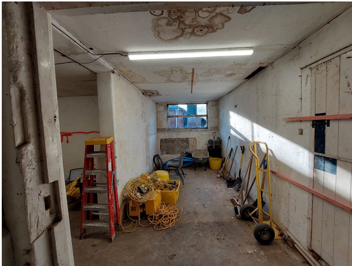
Figure 87: Interior view of the south end of the kennel building.
