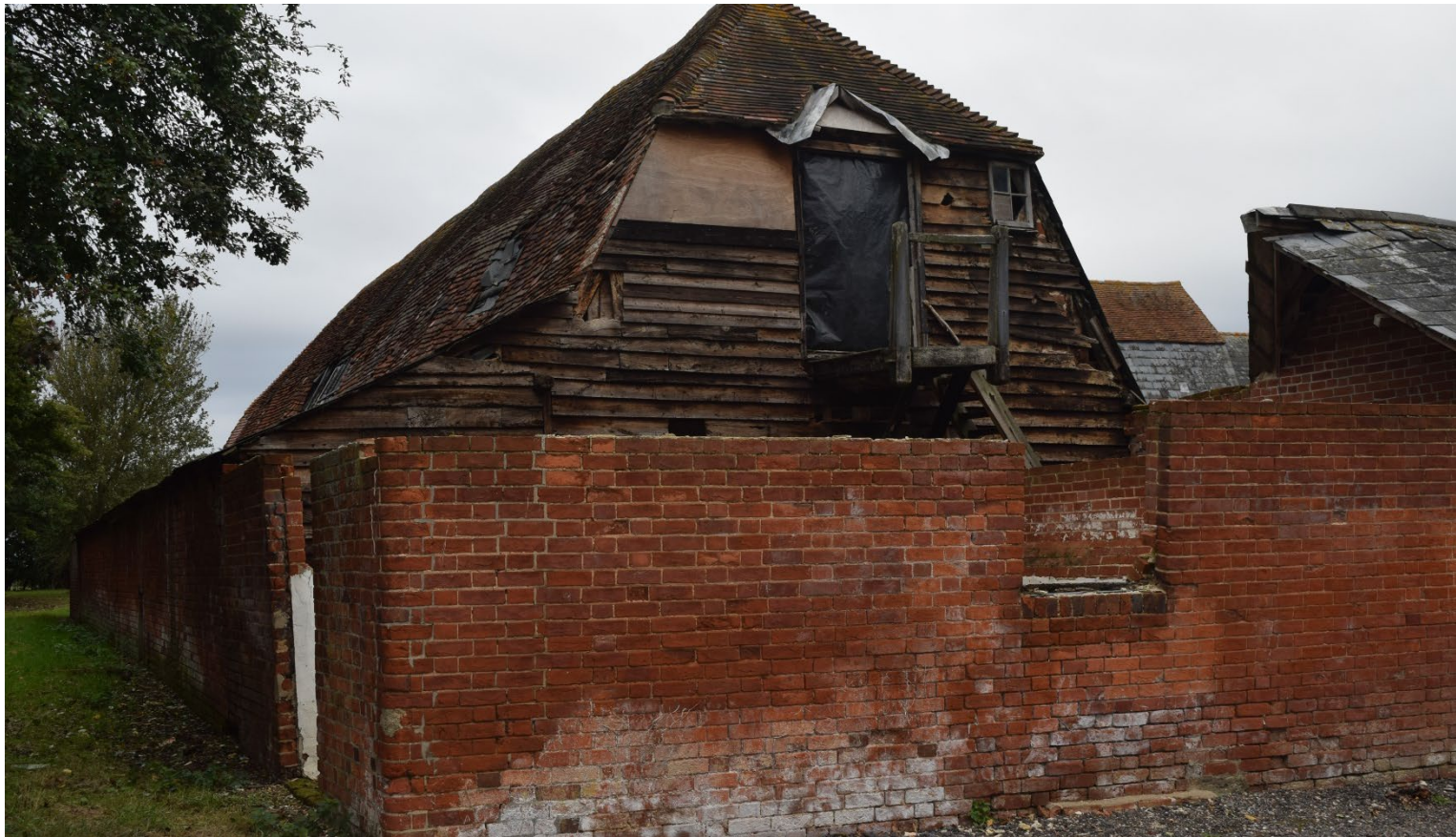
Figure 92: South end range (root house) with inserted doorway into the Byre.
