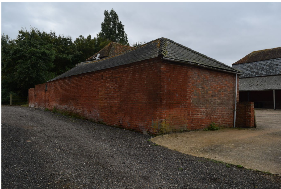
Figure 88: North and East Elevations of the 2-bay open fronted shelter shed.
