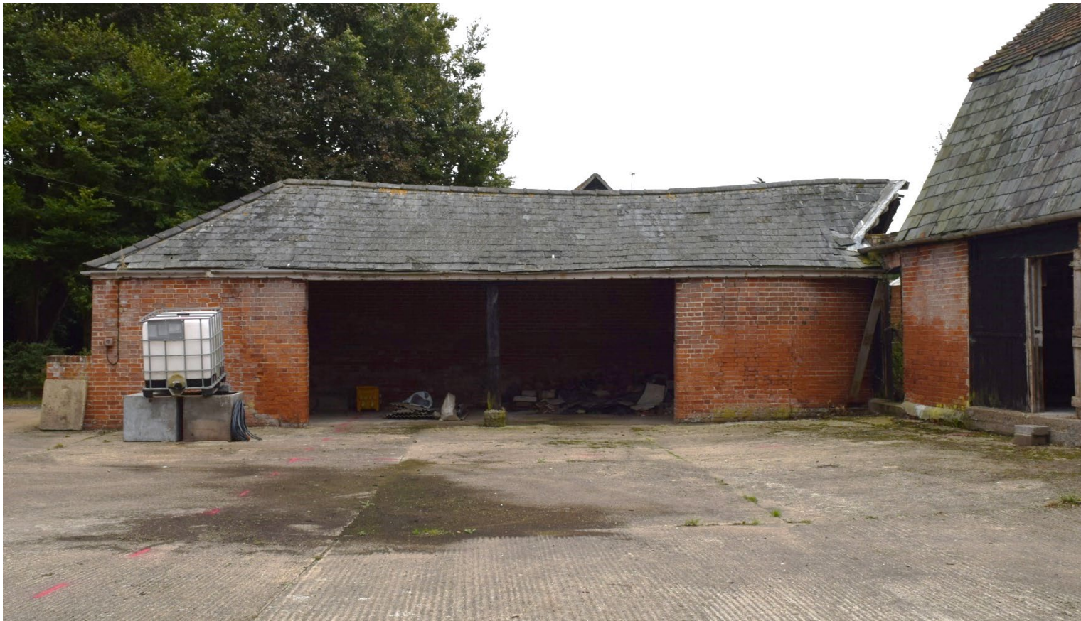
Figure 90: West Elevation of the 2-bay open fronted shelter shed.
