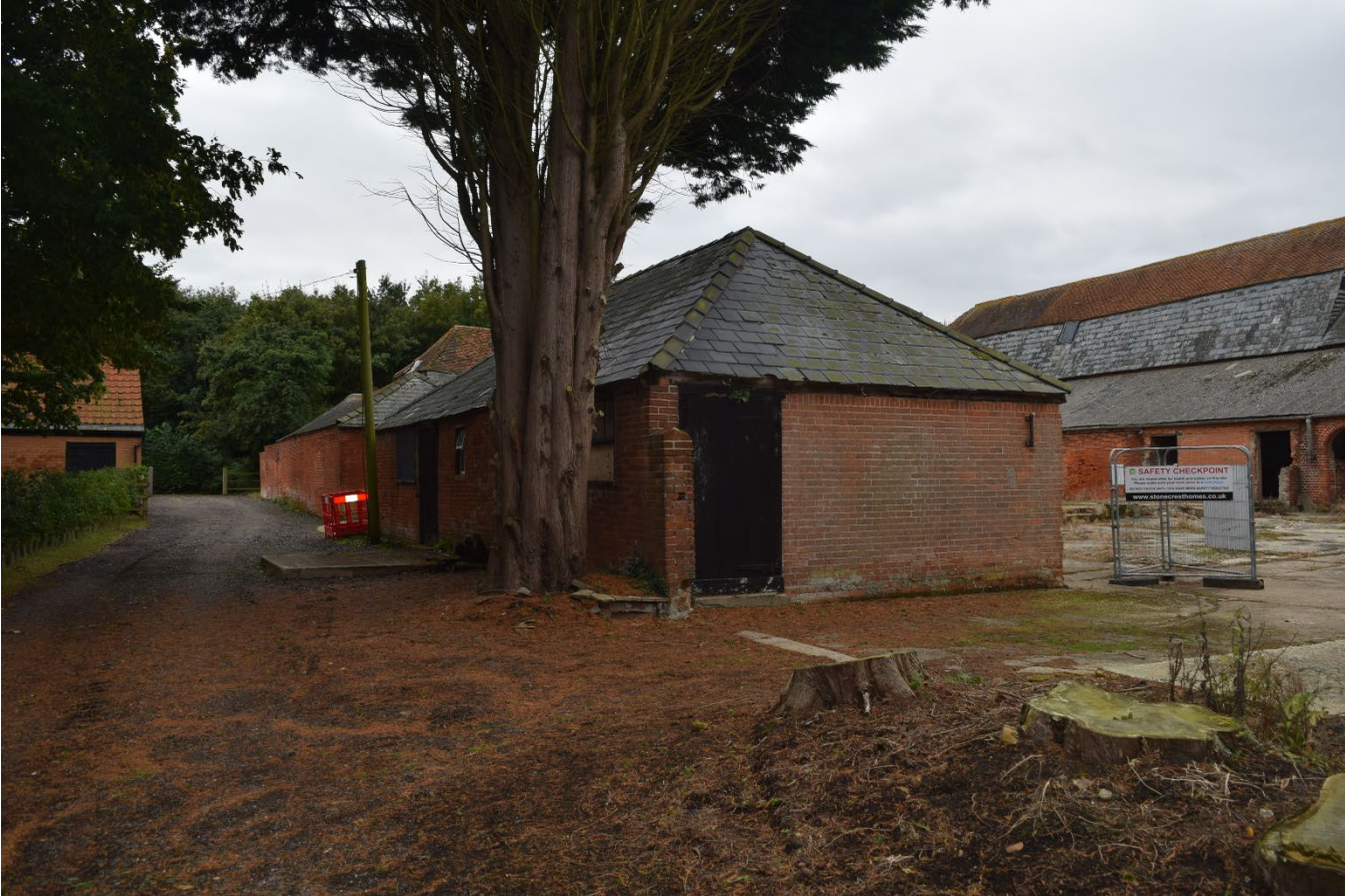
Figure 81: East and North Elevations of the existing Kennel building. Built between 1874-1875.
