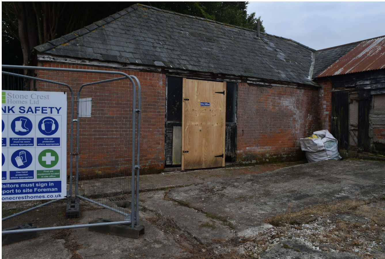
Figure 83: North end section of the Kennel building.
