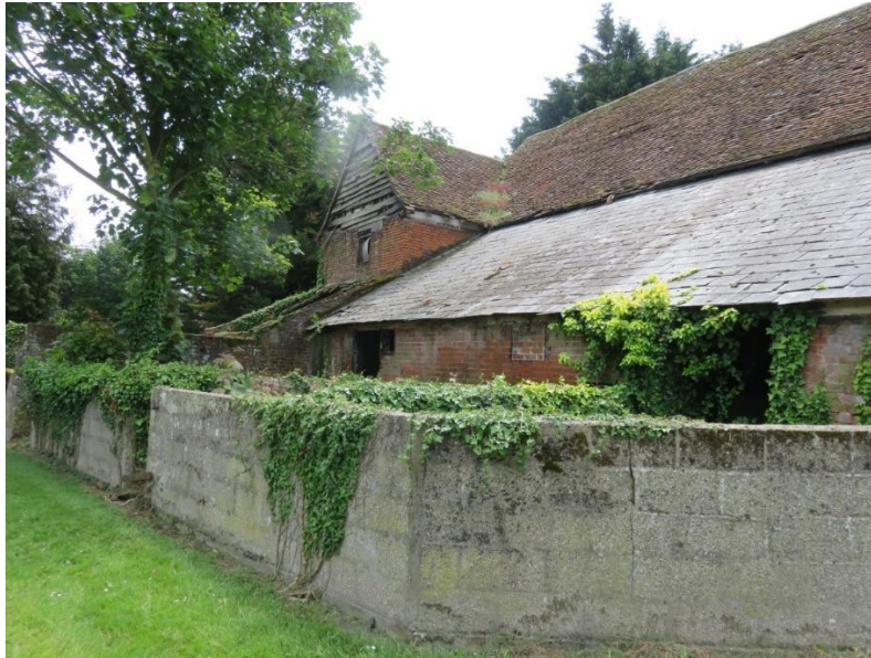
View of lean-to on north side of C17 barn
