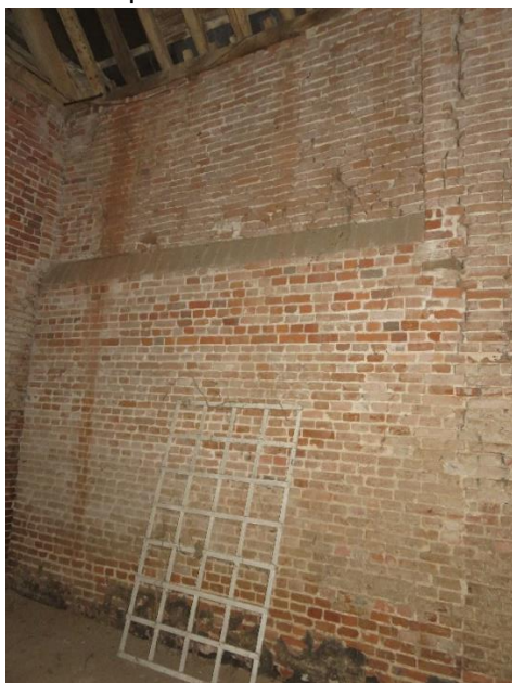
Barn wall south side
