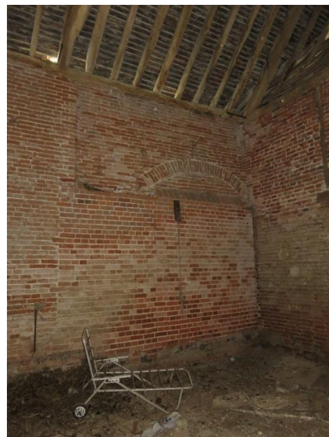
Barn wall north side
