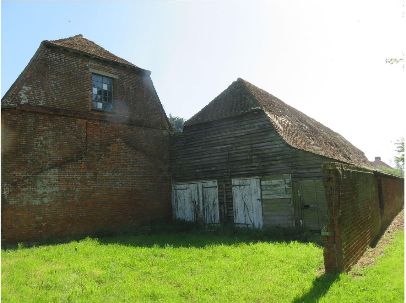
Section of brick wall to be retained to RHS of photo
