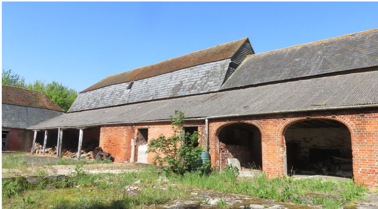
East courtyard elevation of 18 th century barns and lean-to
