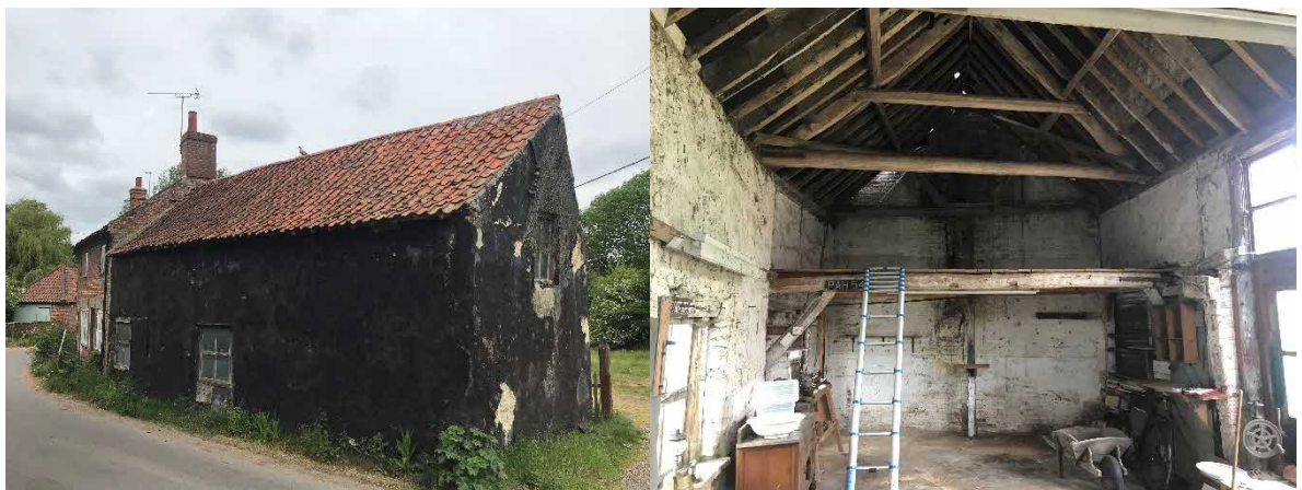
Fig 10 & 11 South and east elevations of barn (left) and internal view (right)
