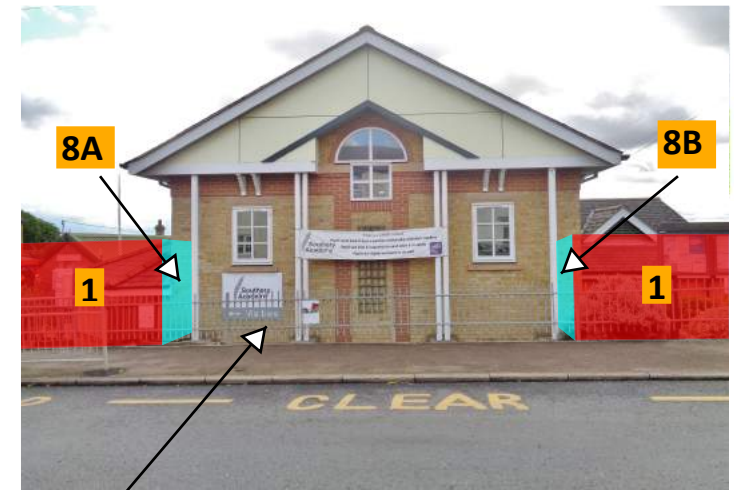
Front of Academy Building adjacent Westgate Street
