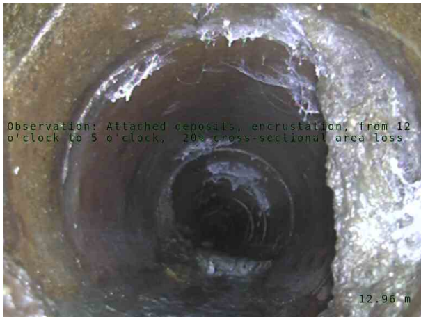
MH01CX_0001.jpg, 00:02:08, 12.96 m Attached deposits, encrustation, from 12 o'clock to 5 o'clock, 20% cross-sectional area loss
