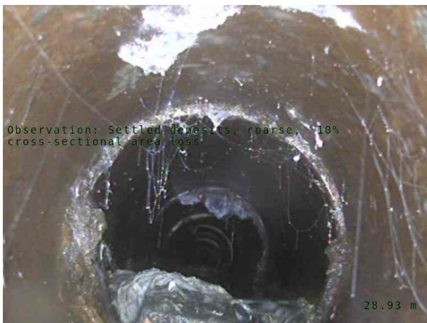
MH01CX_0003.jpg, 00:03:42, 28.93 m Settled deposits, coarse, 10% cross-sectional area loss
