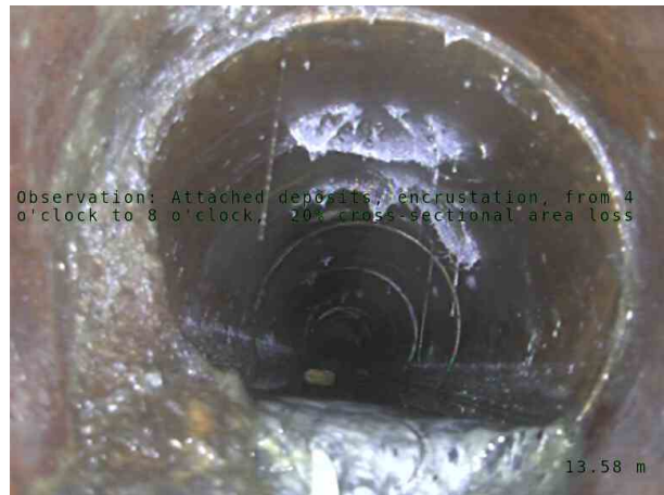
MH01CX_0002.jpg, 00:02:17, 13.58 m Attached deposits, encrustation, from 4 o'clock to 8 o'clock, 20% cross-sectional area loss
