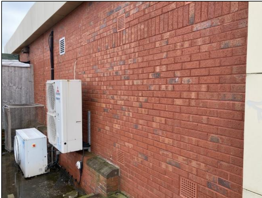
Photograph 10 showing the exterior of the building
