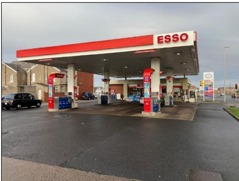
Photograph 14 showing the canopy over the forecourt
