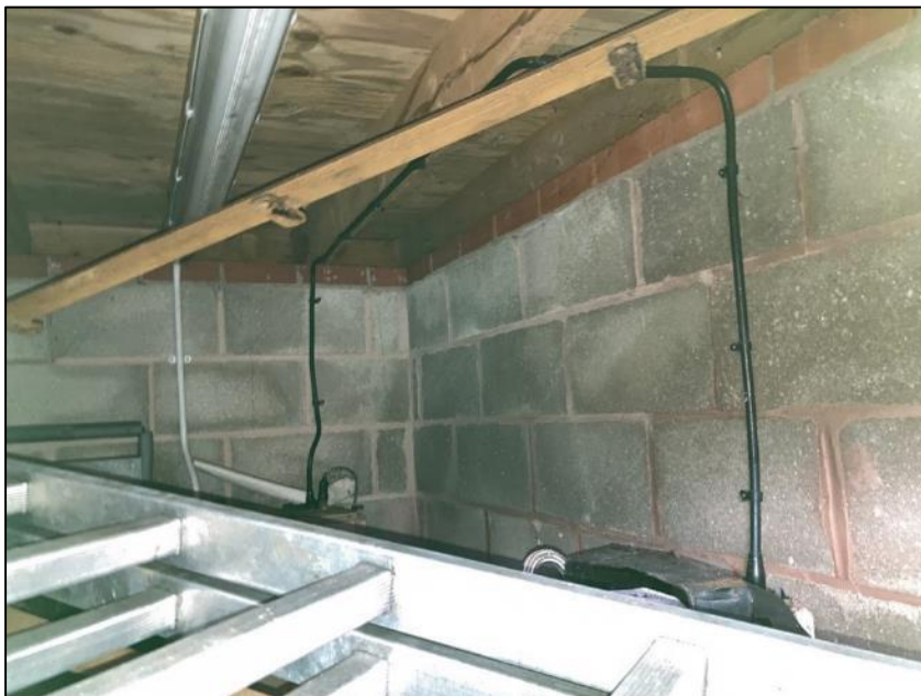
Photograph 22 showing the interior of the storage building
