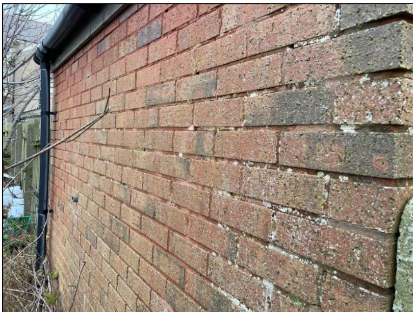
Photograph 20 showing the external masonry
