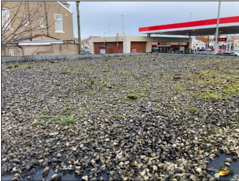
Photograph 21 showing the flat roof
