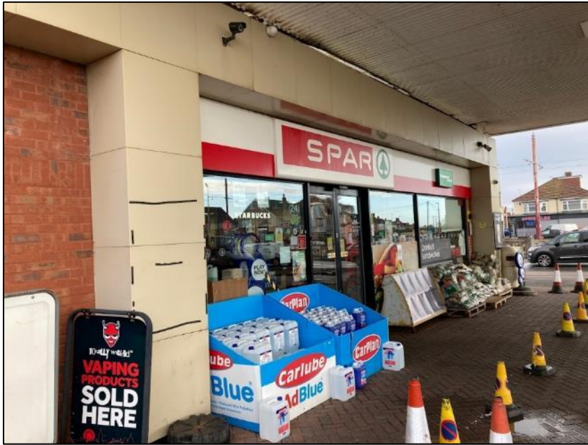
Photograph 11 showing the exterior of the building
