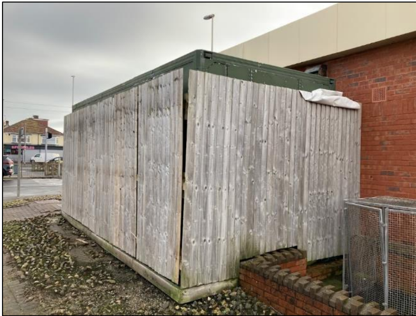
Photograph 13 showing the exterior of the building
