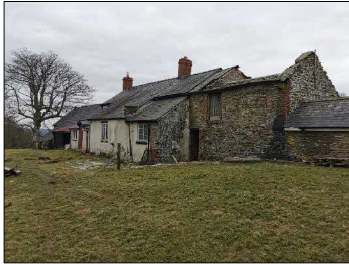
Plate 3. North-western elevation of farmhouse
