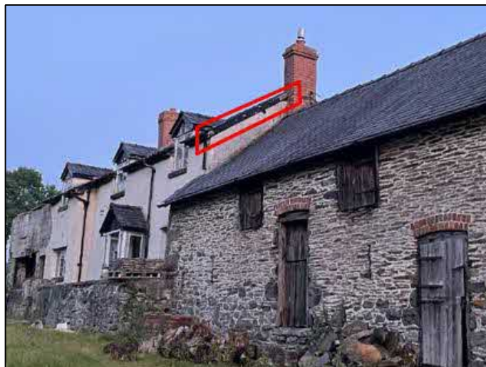
Plate 15. Hole in soffit and under lifted roof tiles
