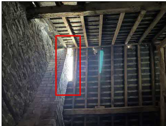
Plate 21. Hole in south-western end of barn roof
