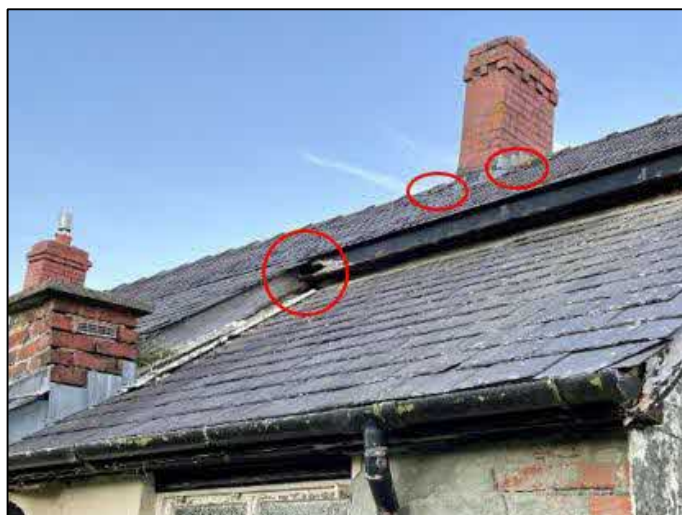
Plate 15. Hole in soffit and under lifted roof tiles
