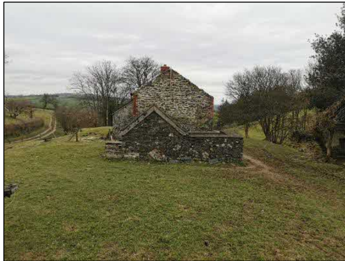
Plate 5. South-western end wall of the stone extension and single-storey pigsty
