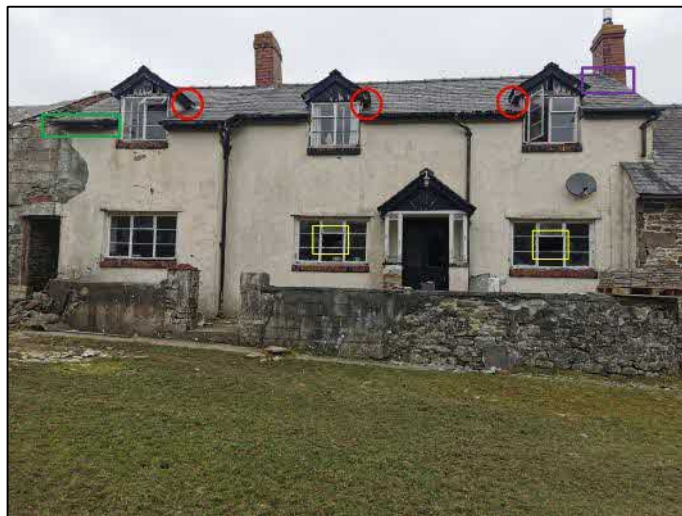
Plate 17. Gaps by dormer windows (red circles), broken windows on ground floor (yellow rectangles), open windows on first floor, gaps at wall top (green rectangle) and lifted tiles around chimney (purple rectangle)
