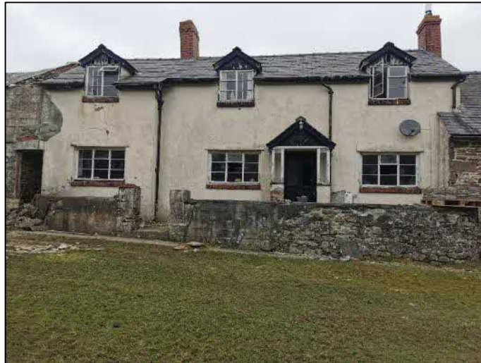
Plate 1. South-eastern elevation of the farmhouse
