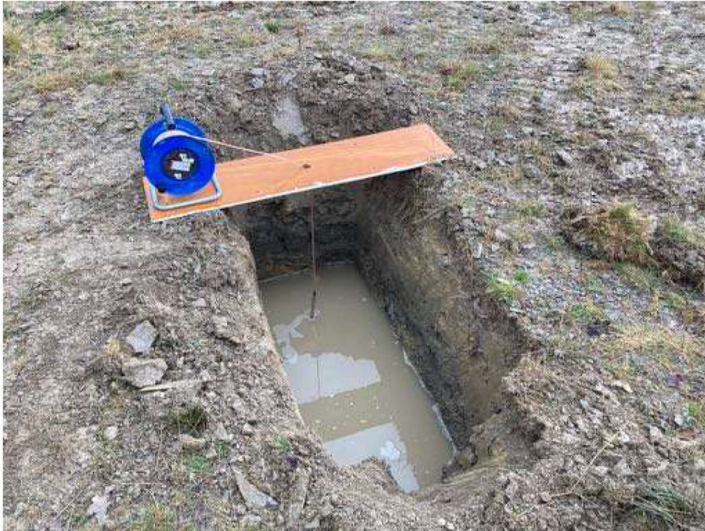
Photograph 13 Description: Water level monitoring at trial pit TP01 (start of test) Date: 28/04/2021 Location: North western part of Site A
