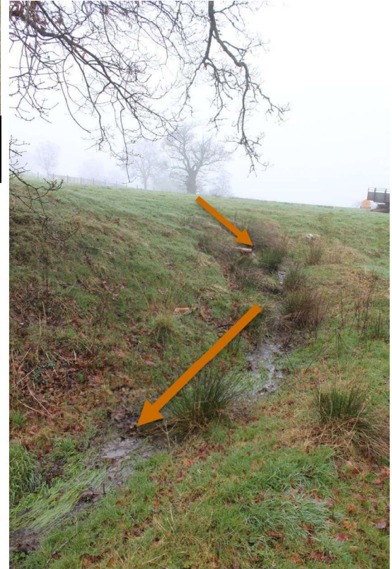
Initial discharge at bottom of field before passing under a track
