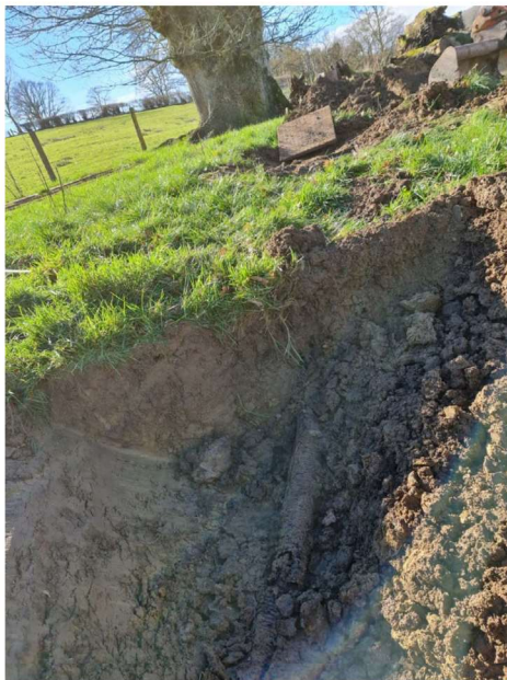
Existing discharge pipe
