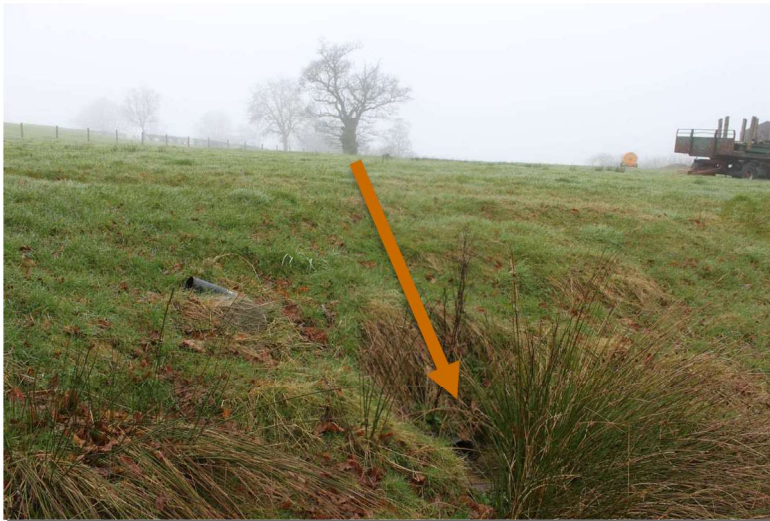
Discharge route down field from receptable (near base of tree)
