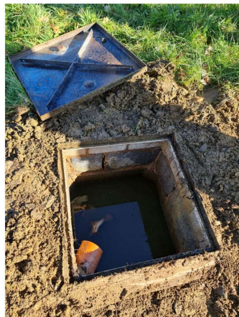
Existing foul water receptacle
