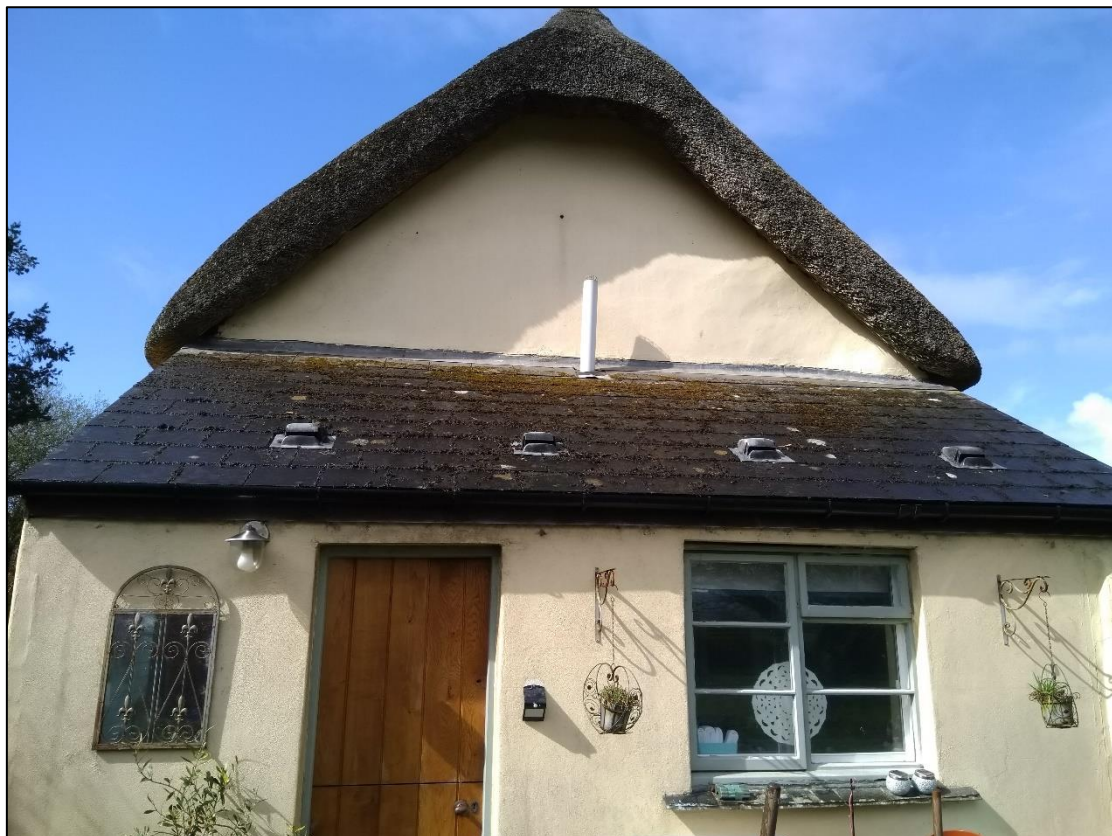
Fig 4 – Existing lean-to extension to northerly gable end.
