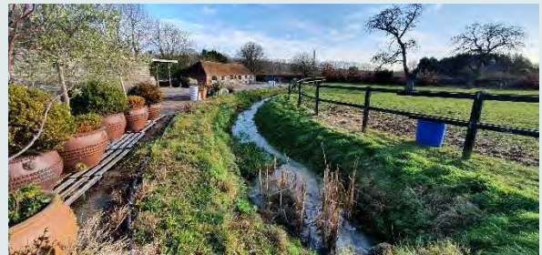
Drainage ditch along southern boundary
