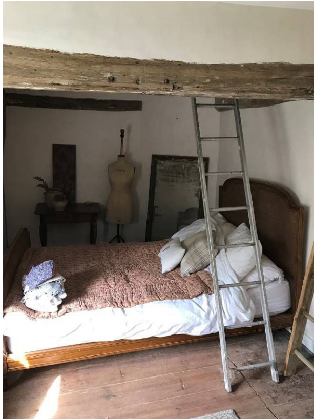
Bedroom 4 – fireplace to be removed & new window opening in back wall
