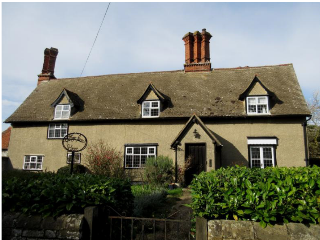
Front Elevation showing existing 20 th Century windows and French doors to be replaced – left-hand windows to be increased in size. Pebbledash render to be stripped off and replaced with lime render.
