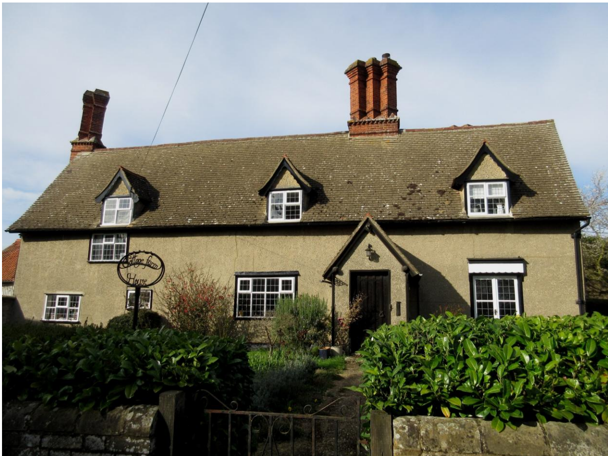
Cottage Farm Buxhall : principal south elevation
