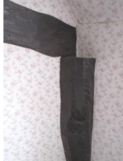
Left: looking N showing door frame let into E tiebeam; Centre: jewelled, adzed SE main post; Right: middle bedroom (W) looking N showing inserted velux and modern cupboards
