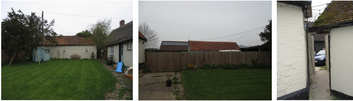
Left: rear garden looking E (building owned by Highams); Centre: looking N towards buildings in separate ownership; Right: passageway, looking SW between house (L) and coal store (R)
