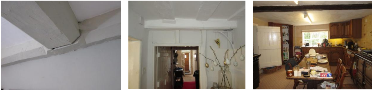
Left: living room axial beam with broad chamfers tennoned into W tiebeam with flat stops; Centre: study (former pantry) looking N through W hall to rear door; Right: kitchen looking S
