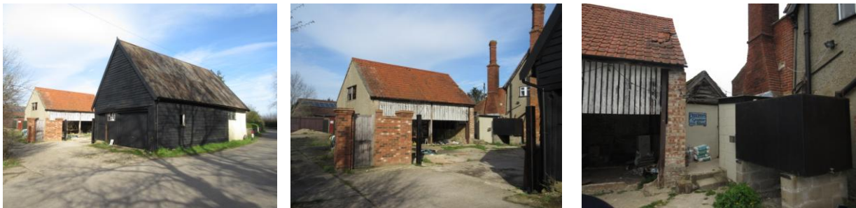
Left: looking N, showing access from Mill Road; Centre: yard and Building B; Right: passageway between Building B and farmhouse, coal store in centre, oil tank on right
