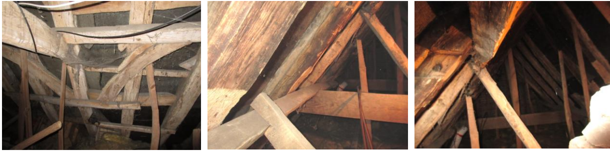
Left: detail of trenched clasped purlin in W section; Centre: looking E into E section towards E gable showing smoke blackening; Right: looking E from N side of stack
