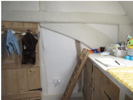
Left: arch brace at N end of tiebeam; Centre: witch marks and rush light burn; Right: W landing
