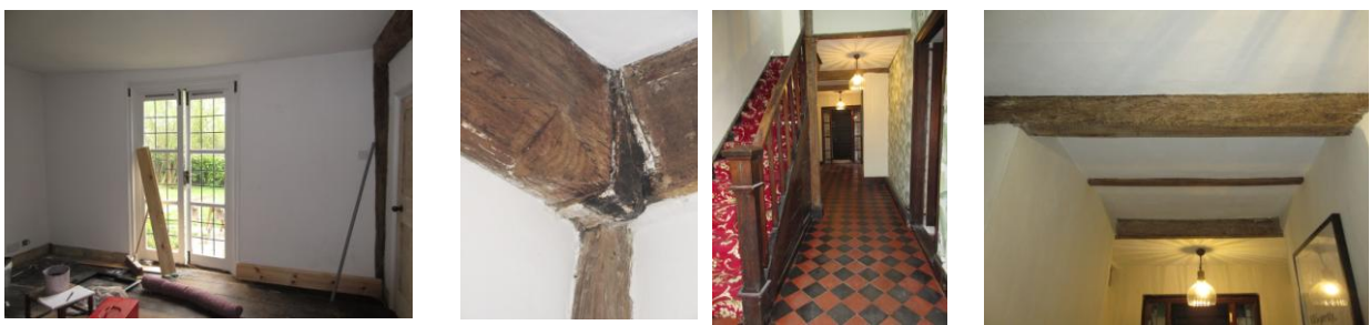
Left to Right: French windows in drawing room; run out stop at N end of chamfered tiebeam above fireplace; stair hall looking S towards front porch; exposed axial beam and joist in hall, looking S
