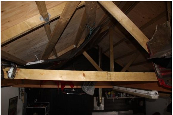
6. Interior of garage
