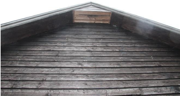
5. Well-sealed boarding at eastern gable
