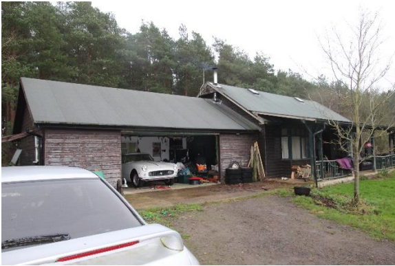
1. Garage and house from the south-west
