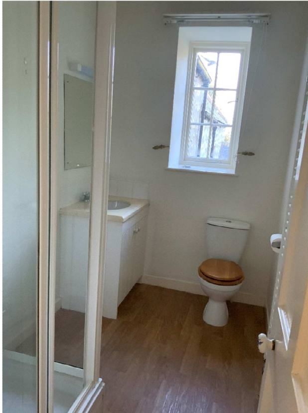
Existing shower room south unit
