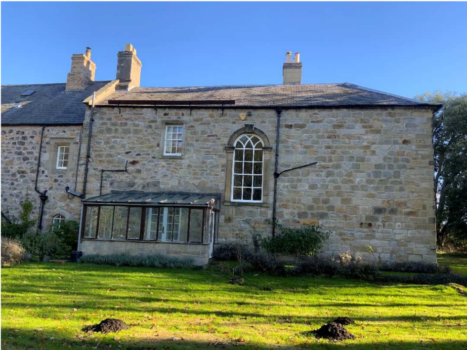
West elevation showing dilapidated conservatory to be demolished
