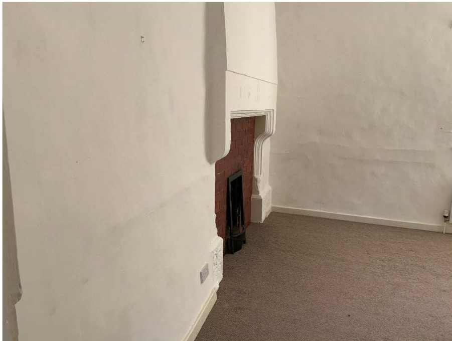
Existing bedroom of north unit unaltered
