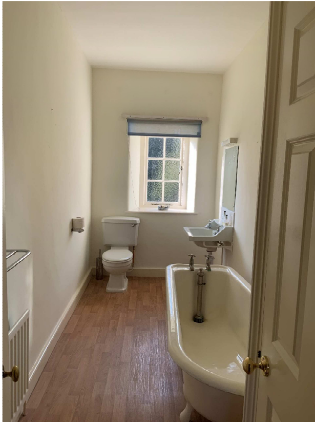
Existing bathroom north unit
