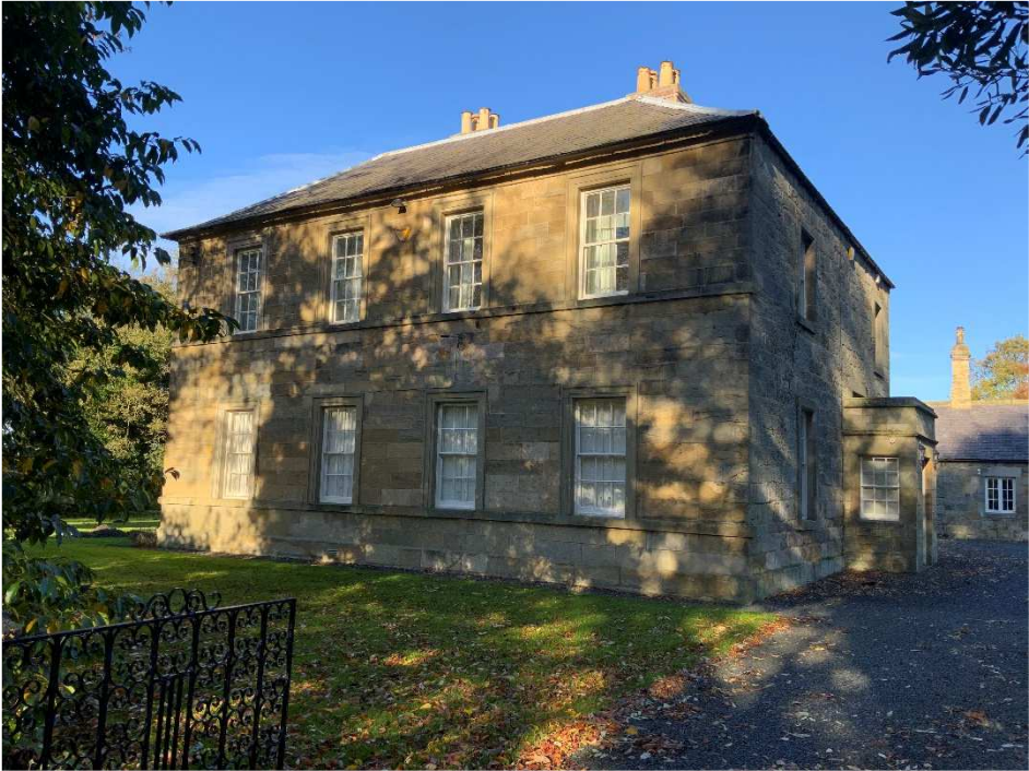
South elevation of south unit
