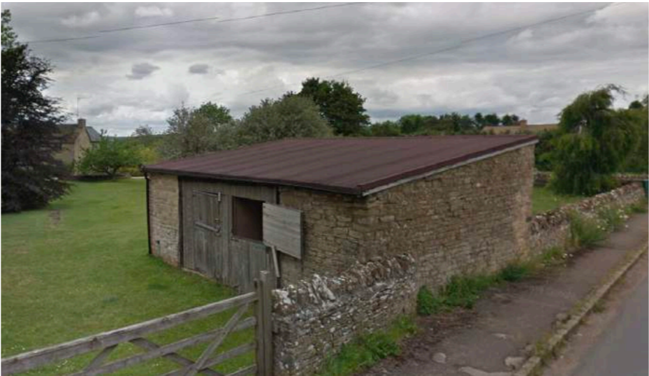
Existing Stables (B)
