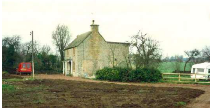
General layout of unauthorised works. Taken 28.11.1987
