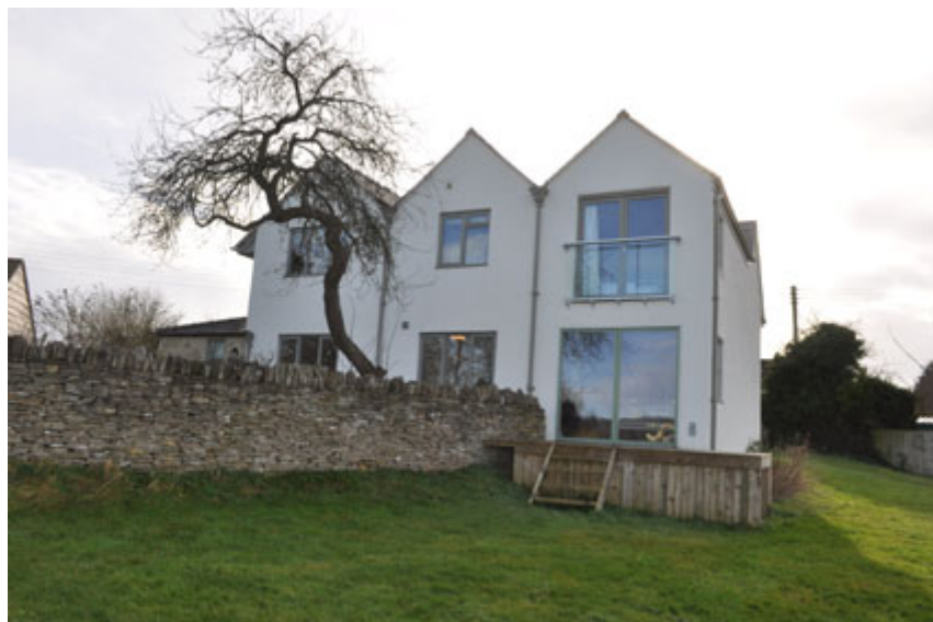
Plate 1: Line of bank and revetting limestone wall
