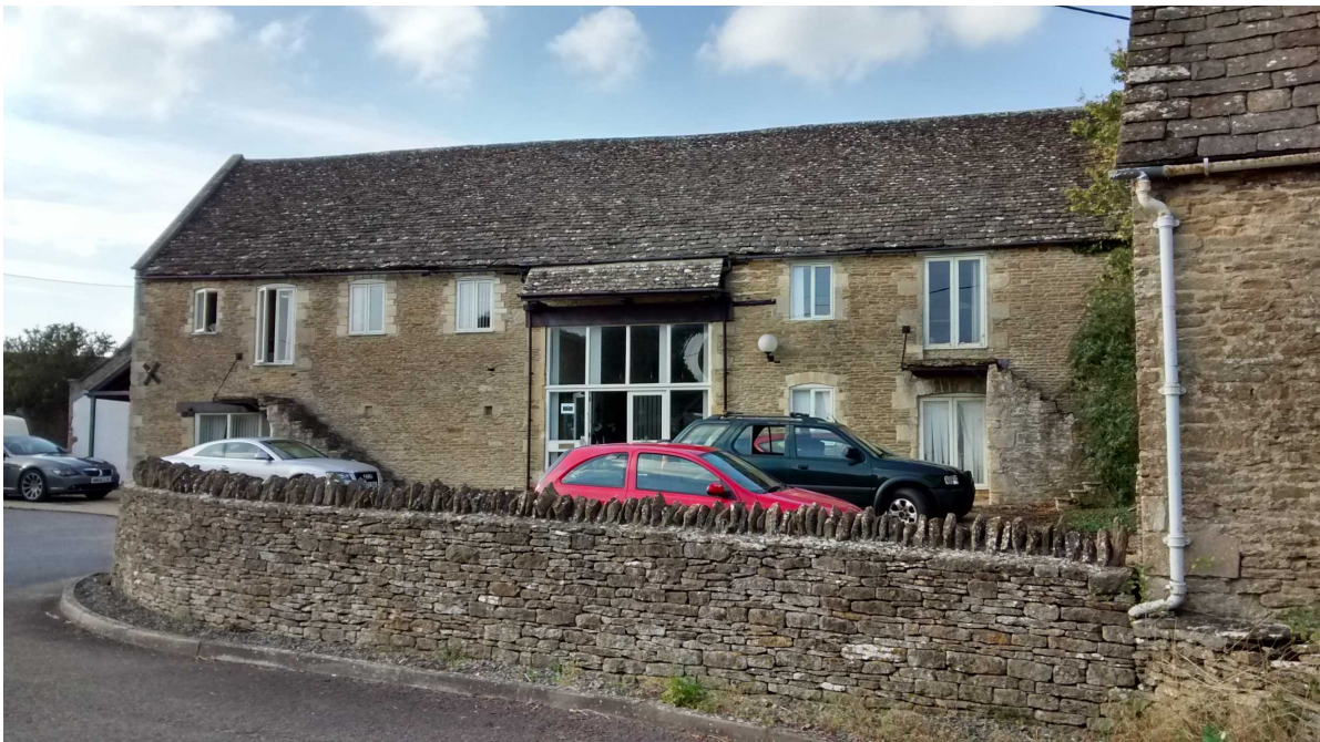
VIEW OF SOUTH EAST ASPECT
