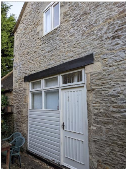
Fig.6 Rear elevation – projecting wing
