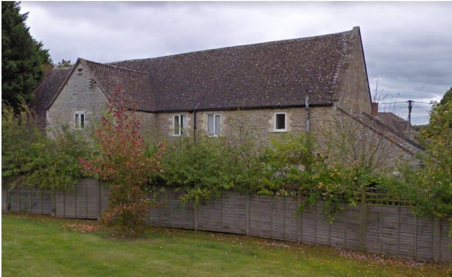
Fig.5 Rear (north-west) elevation
