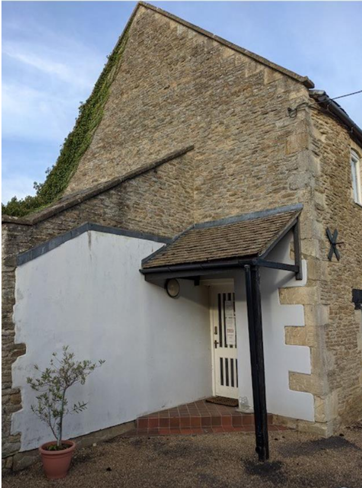
Fig.8 Porch on side (south-west) elevation
