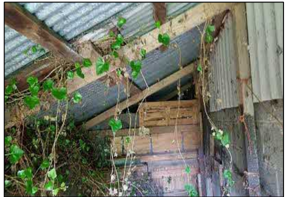
Figure 8: Internal view of lean-to.
