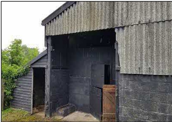
Figure 7: Lean-to next to entrance to rear rooms.
