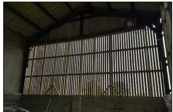
Figure 4: Single ply slatted walls viewed from inside.
