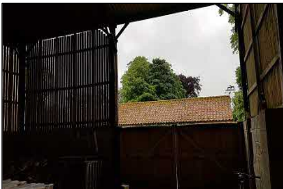
Figure 3: Open fronted barn – viewed from inside
