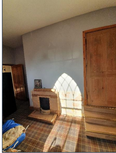
Photo 4 Door and steps in office
