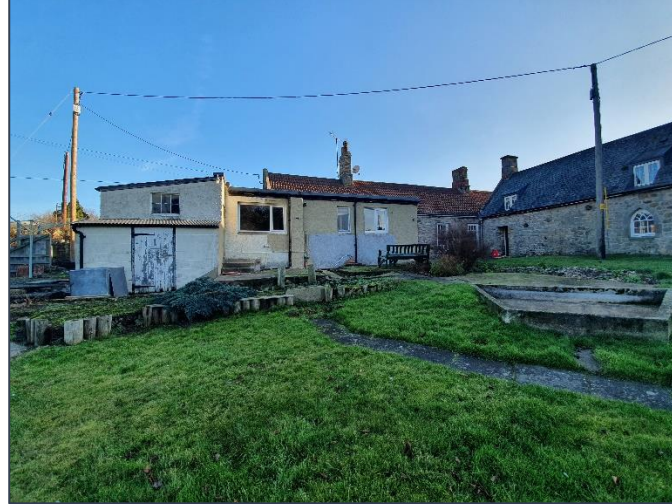
Photo 5 C20th additions of no interest
