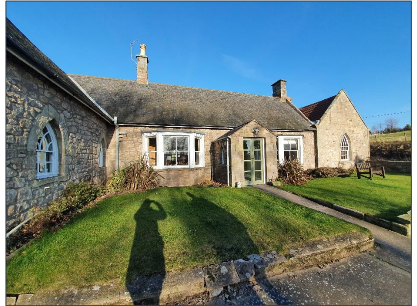
Photo 1 Front south elevation of cottage
