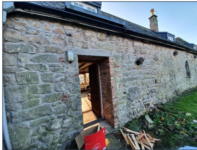
Photo 7 Doorway to north elevation of Reception 2
