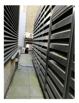
C.2 Photograph of existing acoustic louvred enclosure (existing plant to be removed)
