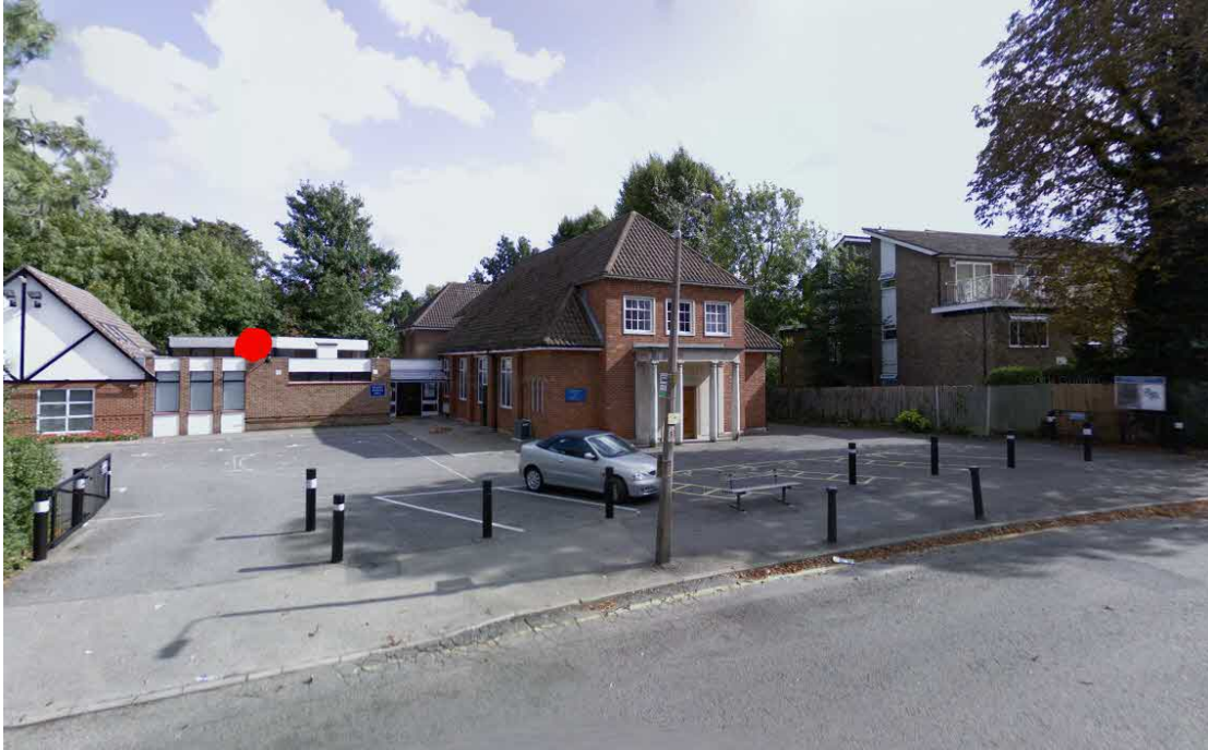
Image of site prior to works progressing, showing approximate location of extract fan.
