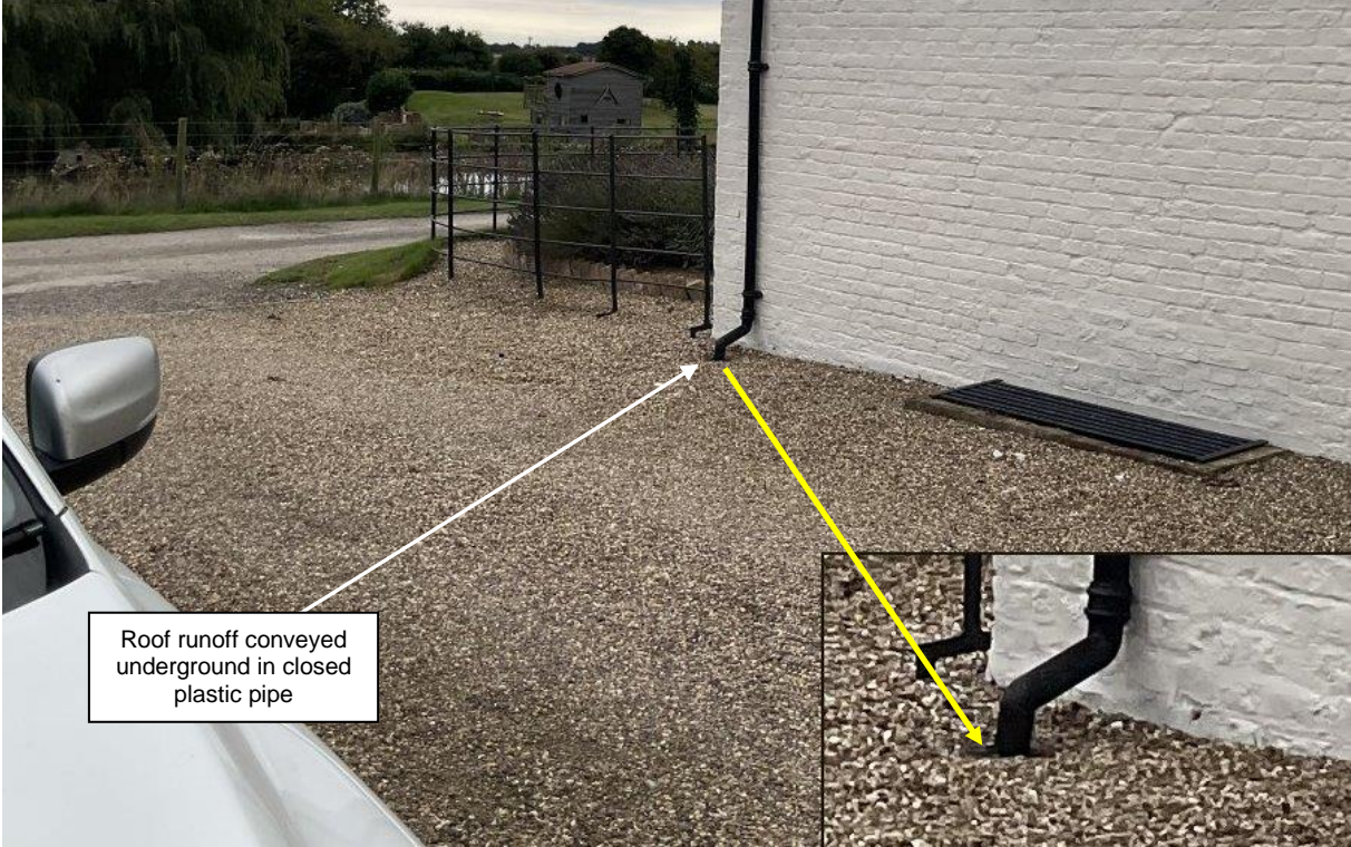
Figure 16 Roof runoff at the farmhouse, adjacent to the access road
