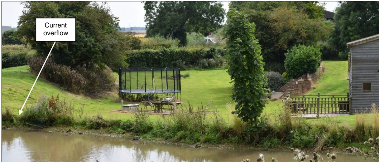
Figure 22 Outflow and emergency overflow route from the attenuation pond
