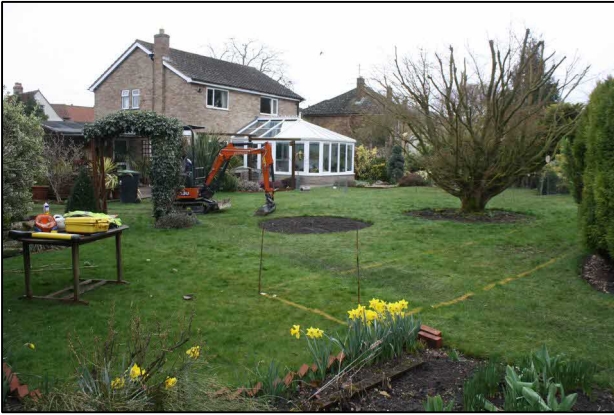
1 View of site before excavation of trench
