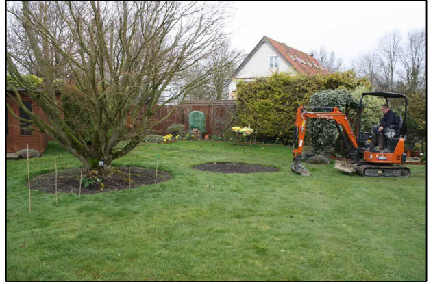
2 Trench being excavated
