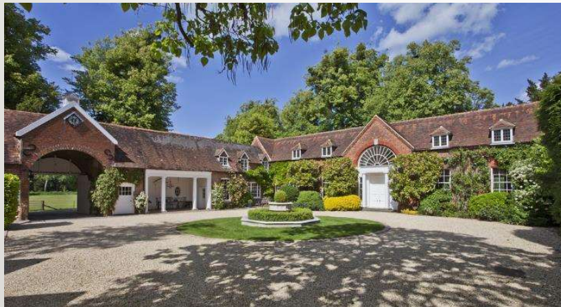
Stable block courtyard
