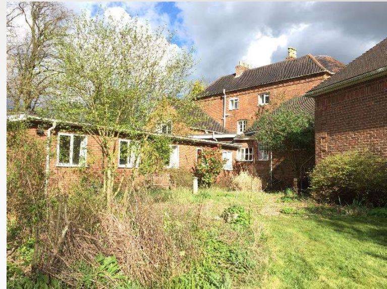
West elevation of Offa House concealed by awkward modern additions
