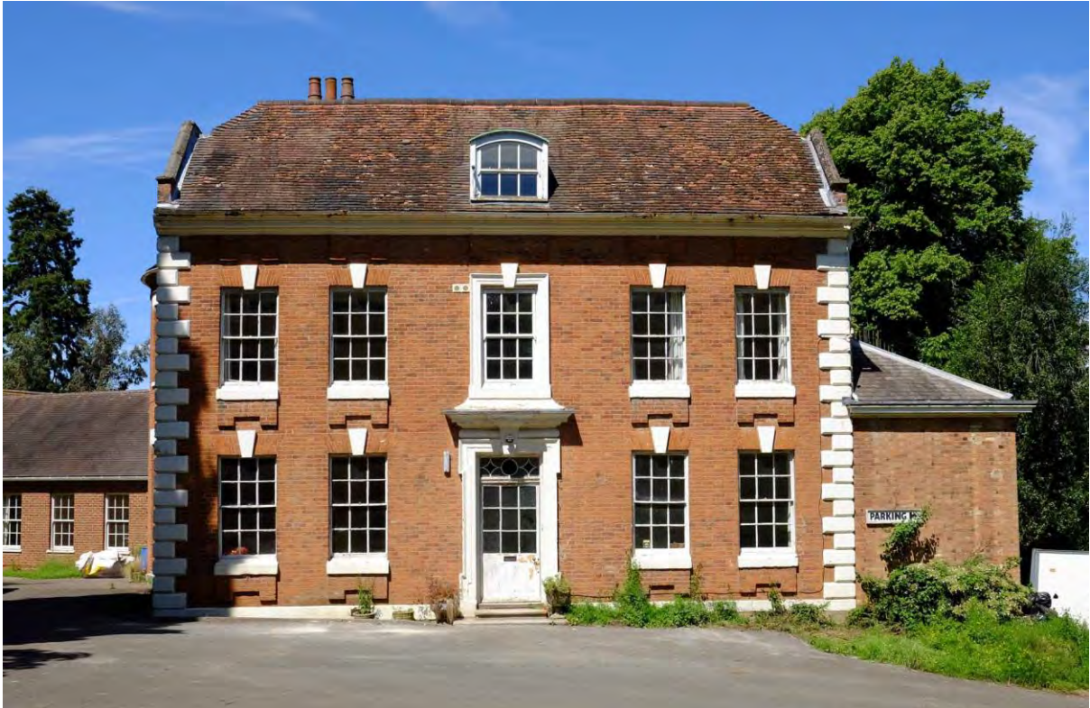
1: Offa House principal elevation
