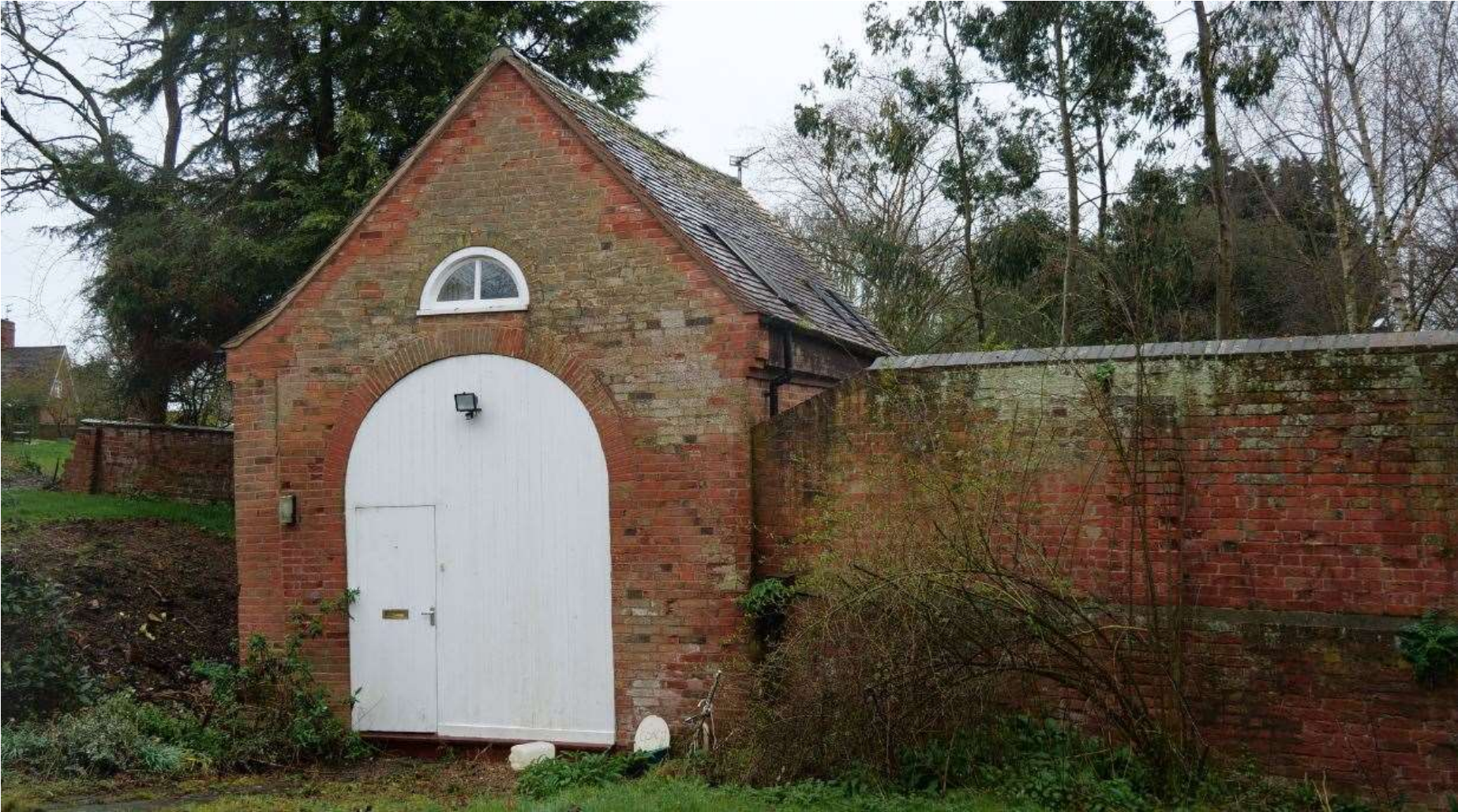
Figure 15: View of 'Coach House' frontage with associated wall
