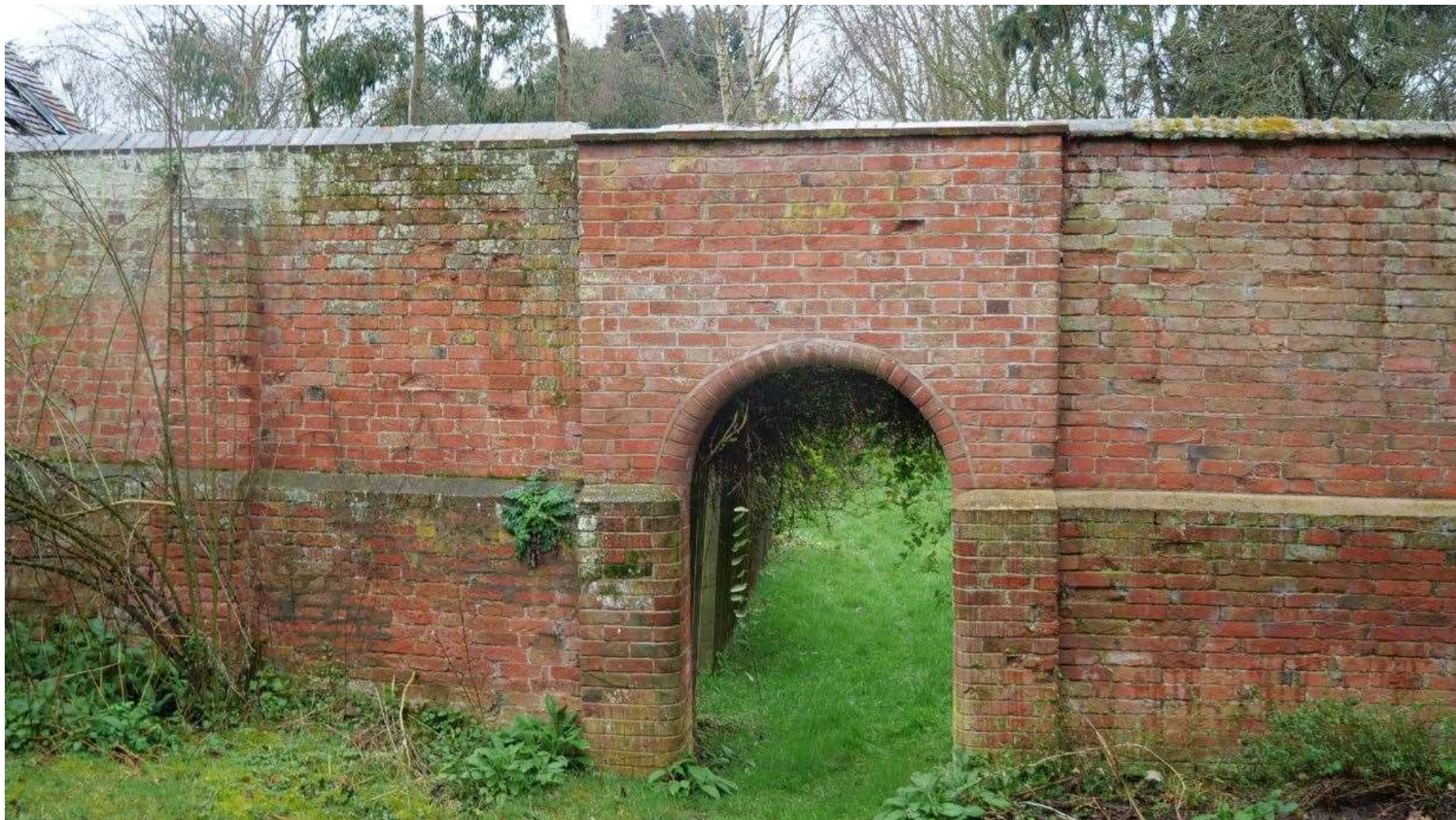
Figure 16: View Northern Side of Wall and later inserted arch
