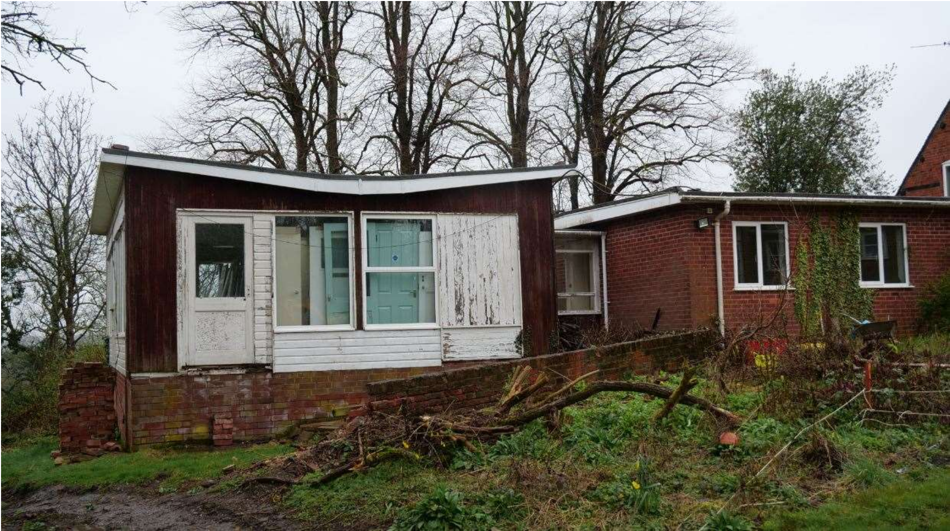
Figure 19: View of C20 Wing from Southern Side
