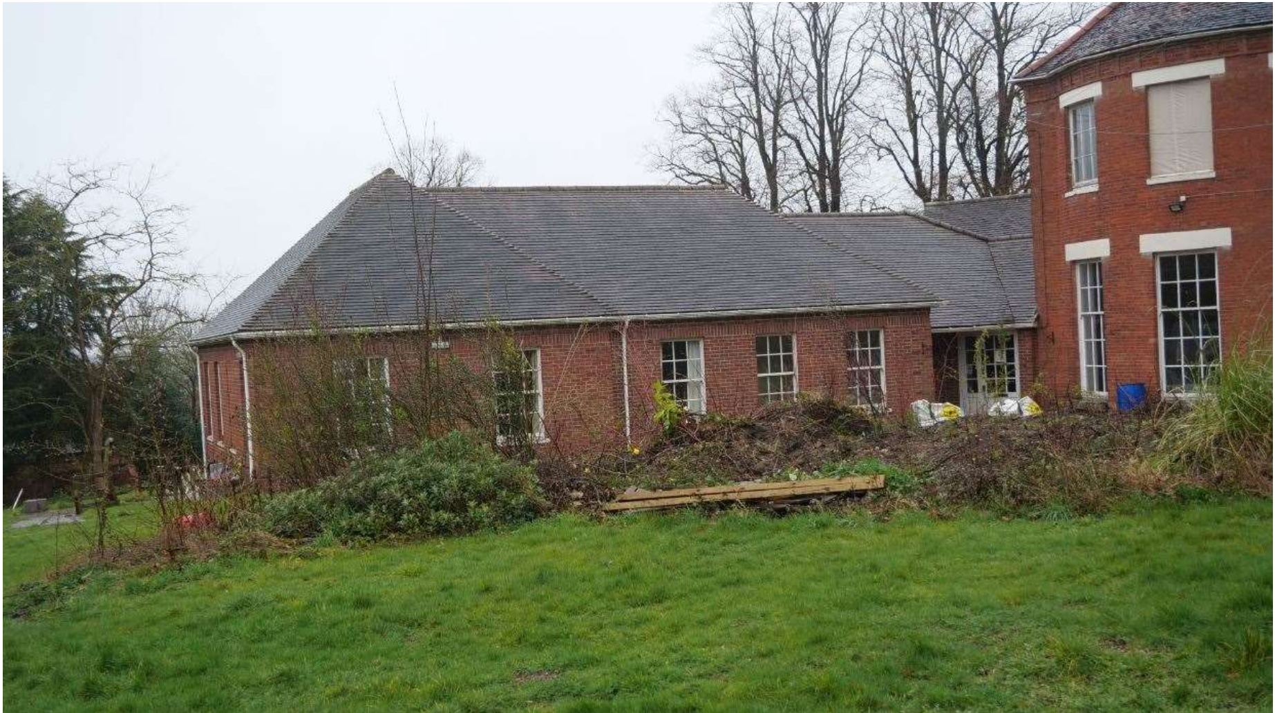
Figure 22: View of South Elevation of Offa House and 1980's Wing
