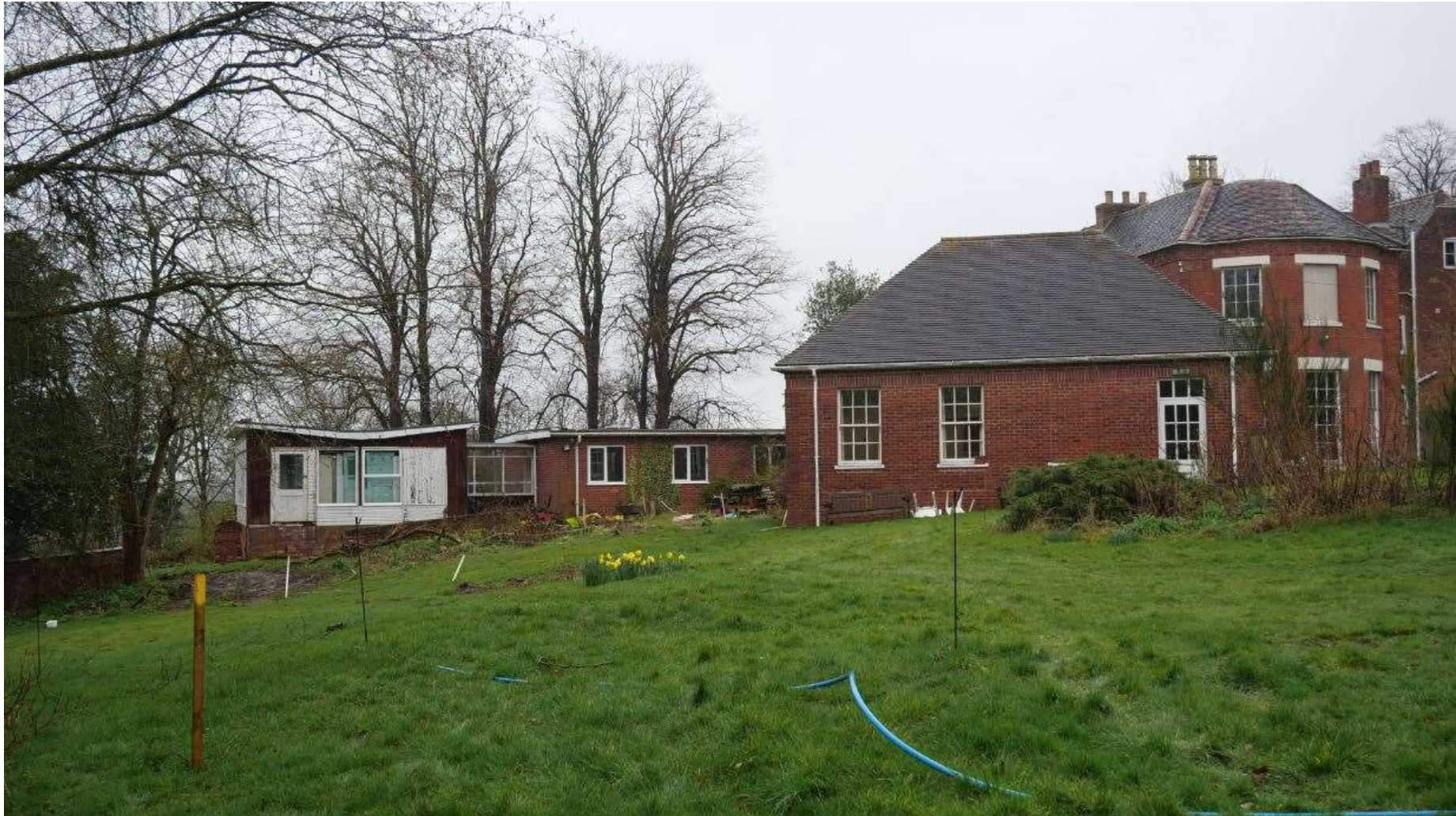
Figure 21: View of South Elevation of Offa House, 1980's Wing And C20 Wing behind
