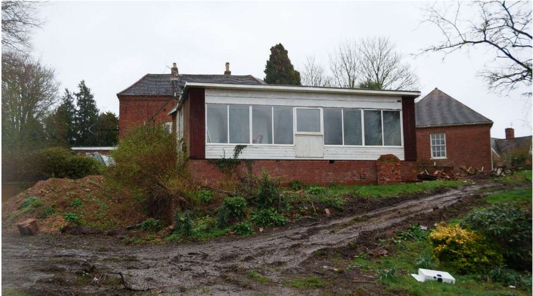
Figure 13: View of Offa House C20 East Wing (South Elevation) with 1980's Wing to right and Lodge Cottage behind
