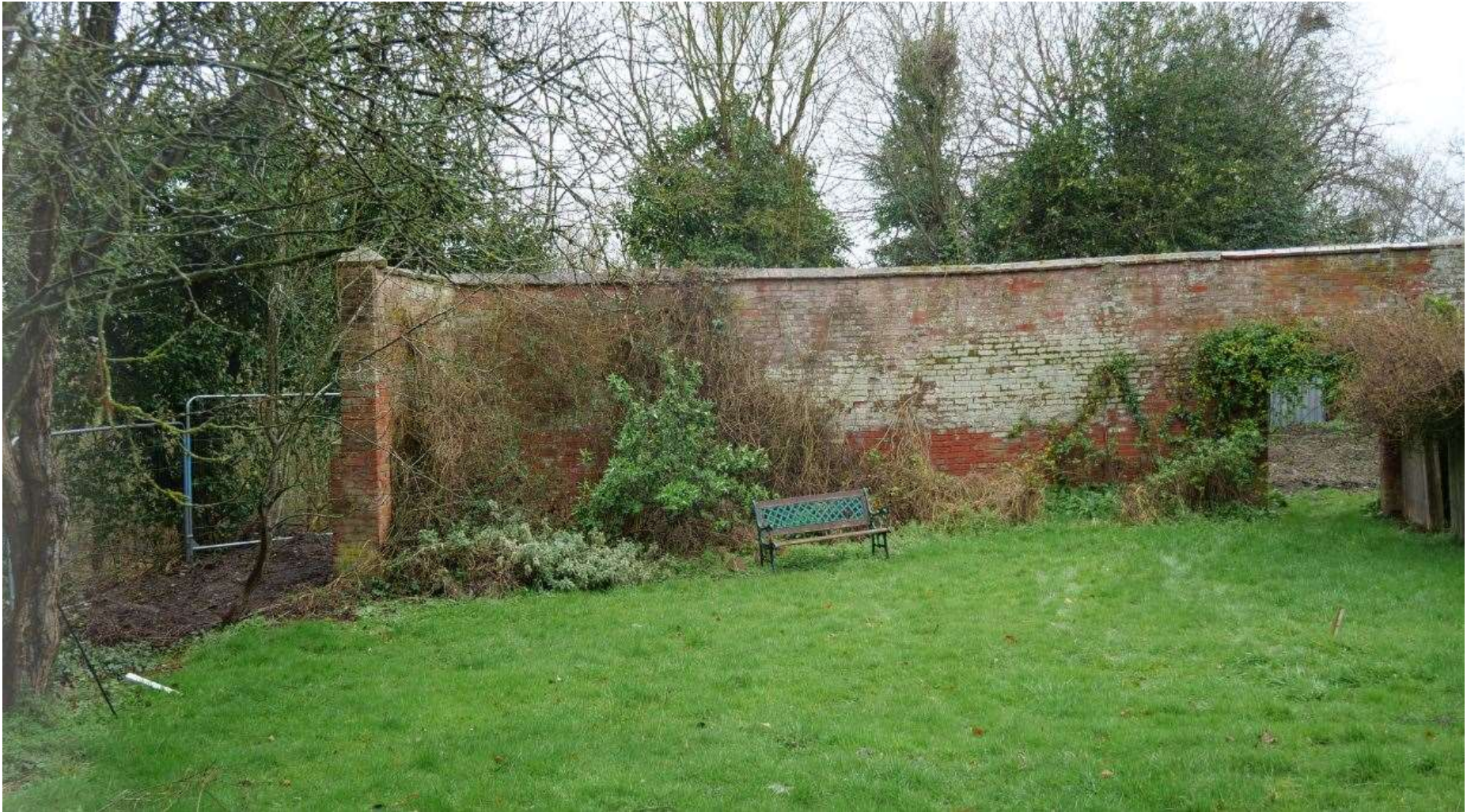
Figure 17: View of Wall from South
