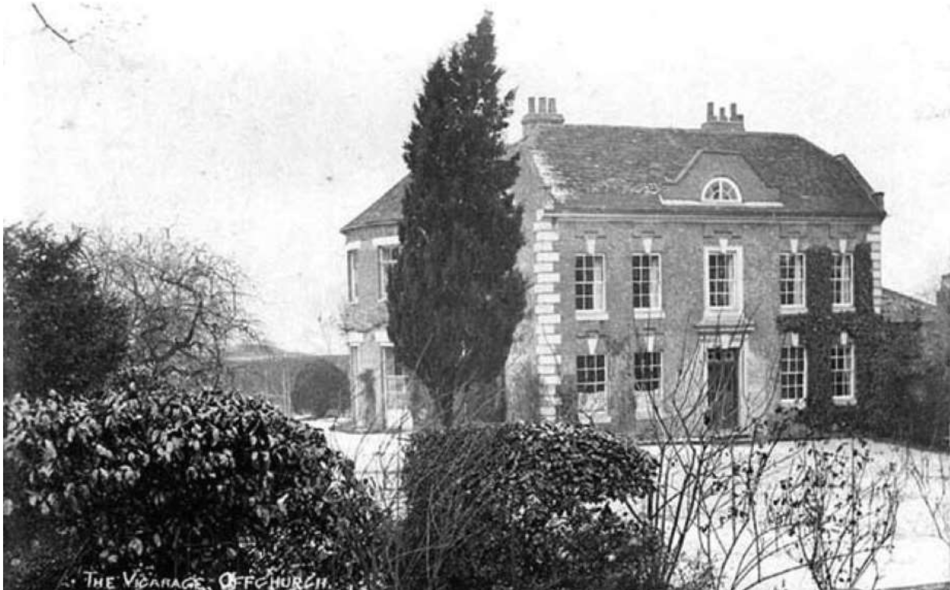
Figure 37: Photograph early C20 – Note earlier three attic dormers seen in 1829 image replaced by new single half round window (now replaced by single dormer window – see Fig. 12)
