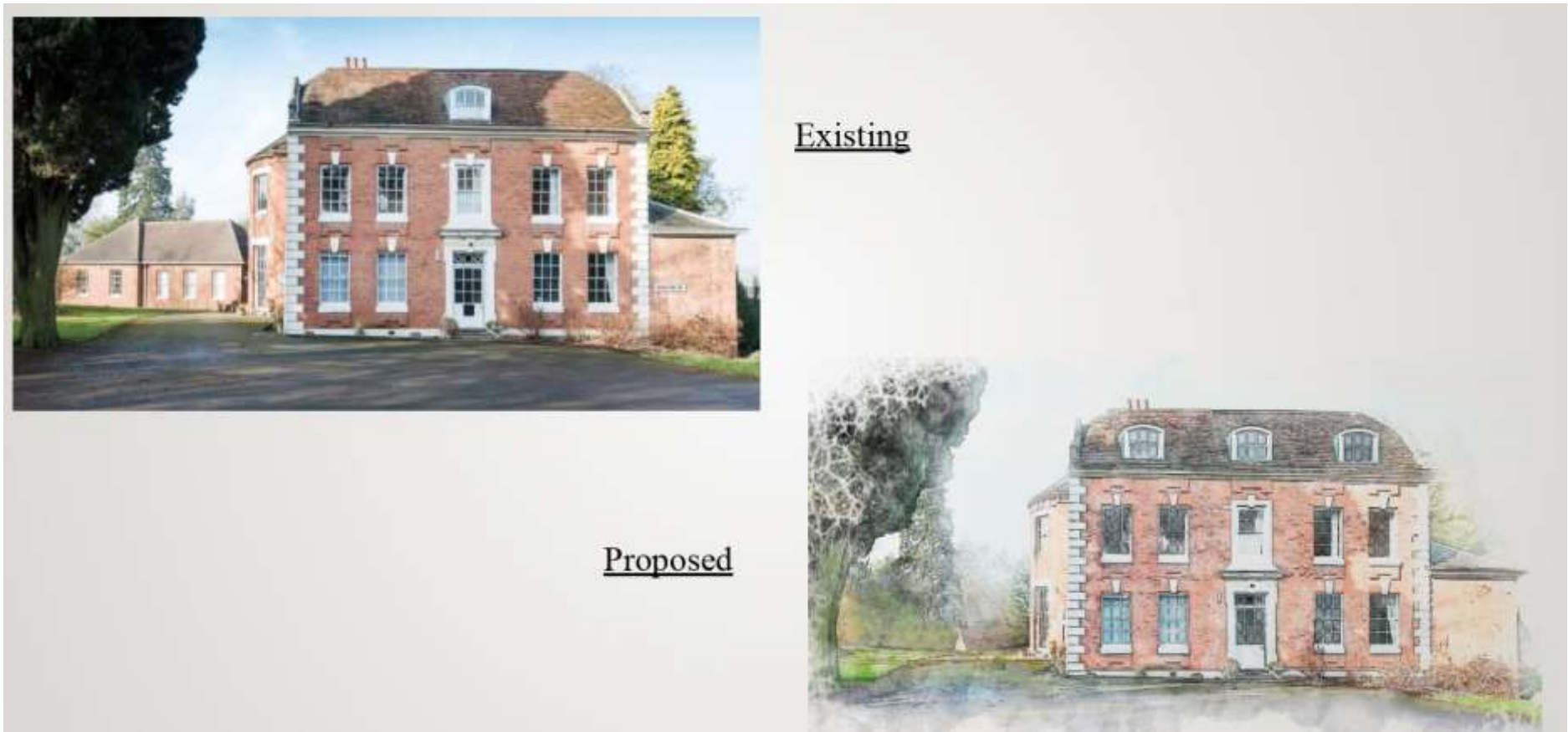
Figure 46: Existing and Proposed Principal Elevation of Offa House (with 3 attic dormers as per 1829 image)
