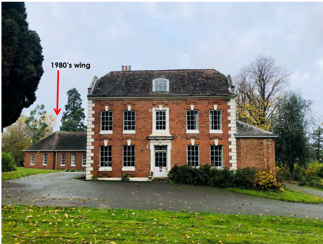
The principal elevation of the property (East elevation)
