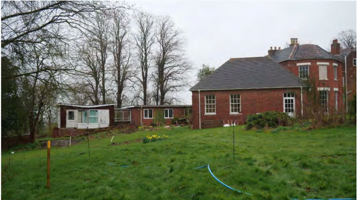
Side (South elevation) showing 20th Century extensions
