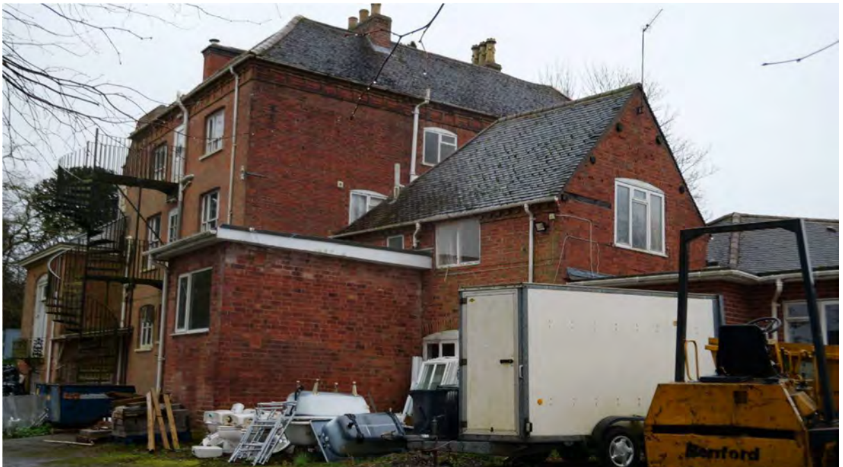
Side (Northern elevation) showing 20th Century extensions and spiral stair case.
