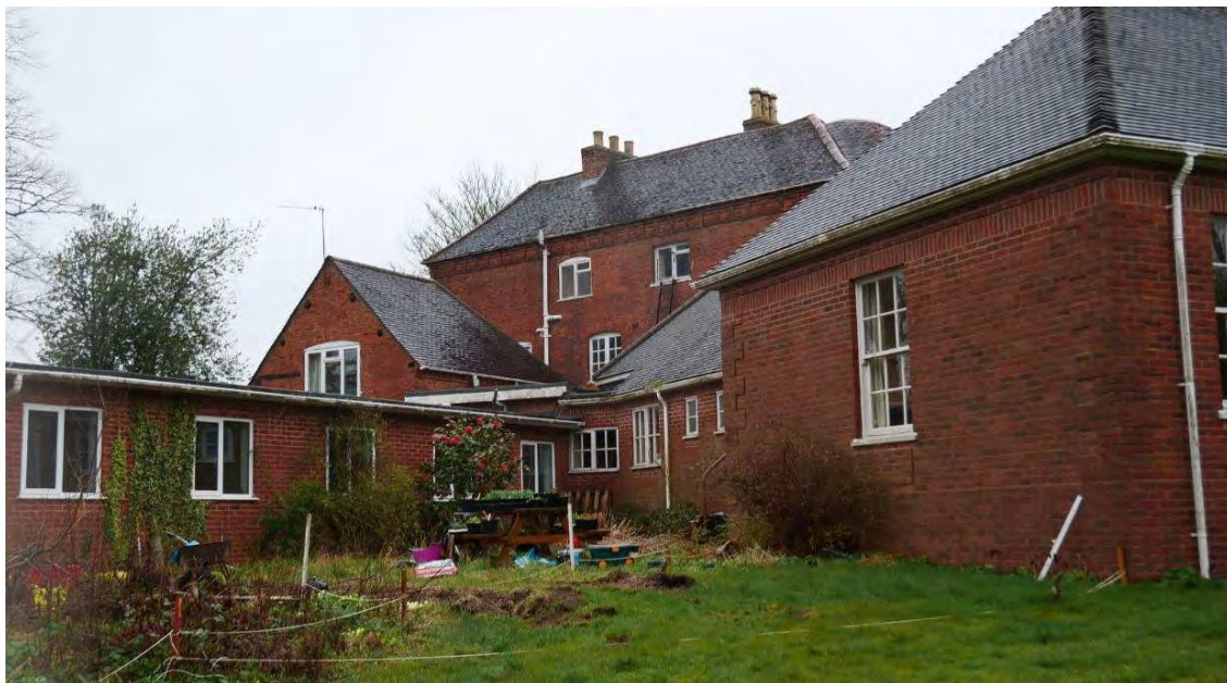
The rear of the property (West elevation) showing 20 th Century extensions
