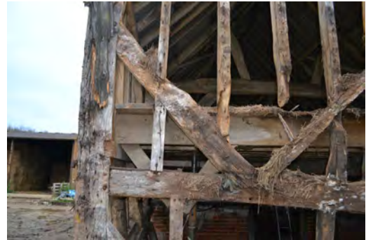
P8 Post mid-rail (Grid A1)
