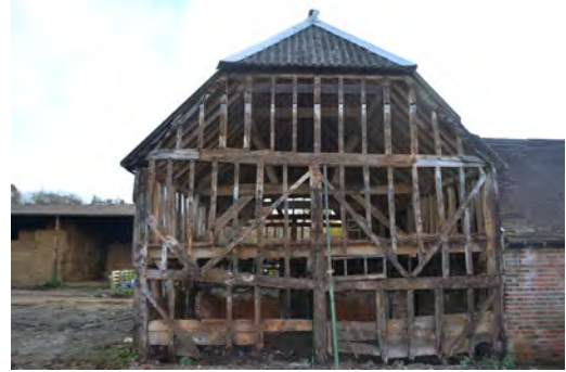
P2 West elevation (Grid 1)
