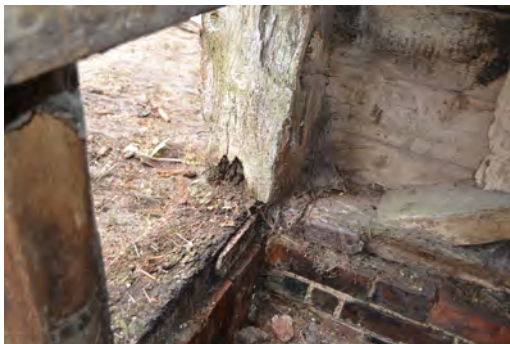
P66 Post base (Grid A7)
