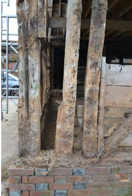
P87 Post base (Grid A9)
