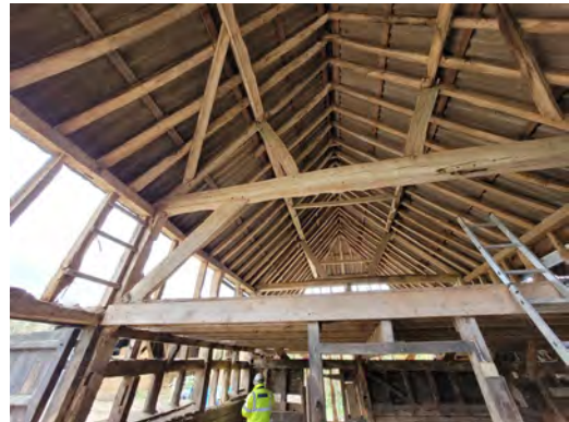
P6 West elevation (Grid 5)
