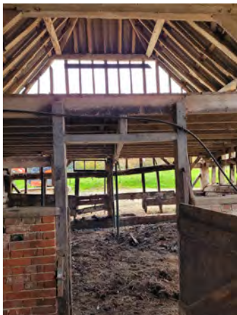
P39 Spine floor beam (Grid B4)
