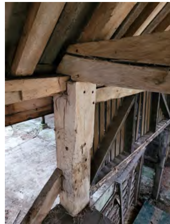
P49 Post to tie (Grid C5)
