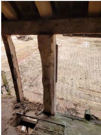
P60 Post to eaves (Grid A6)
