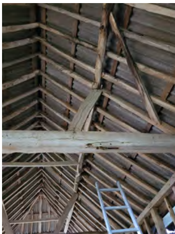
P50 Tie hole for brace (Grid C5)
