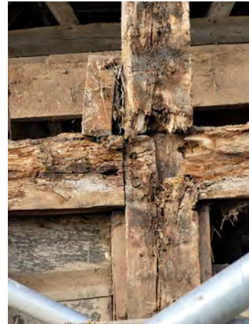
P96 Mid-rail (Grid B9)
