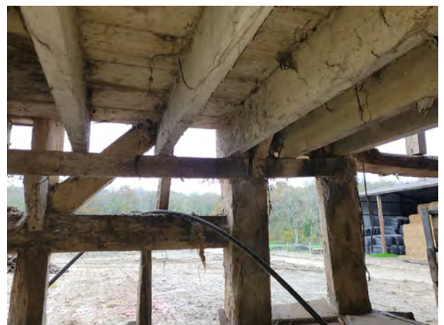
P34 Floor support (Grid A3)
