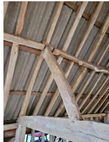
P72 Purlin strut (Grid C7)
