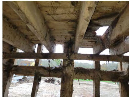
P22 Floor support (Grid A2)
