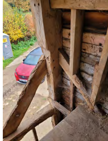
P102 Mid-rail and brace (Grid C9)
