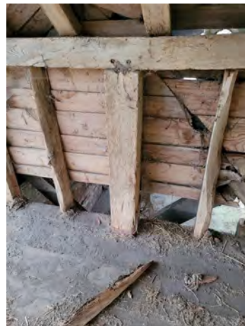
P86 Eaves beam (Grid C8)
