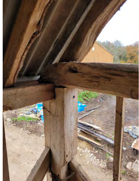
P92 Tie and eaves (Grid A9)
