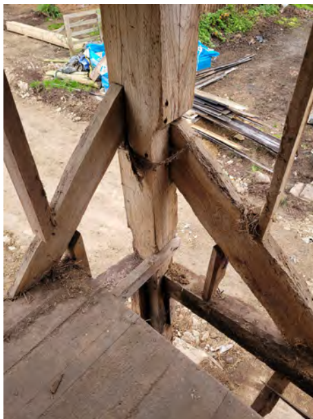
P93 Mid-rail (Grid A9)
