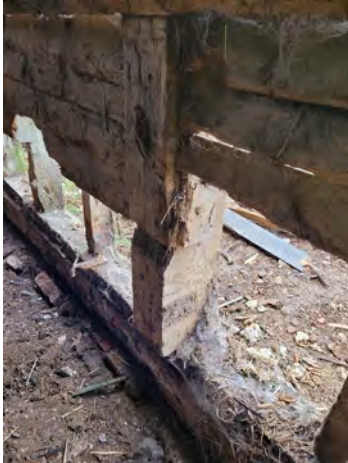
P58 Post base (Grid A6)
