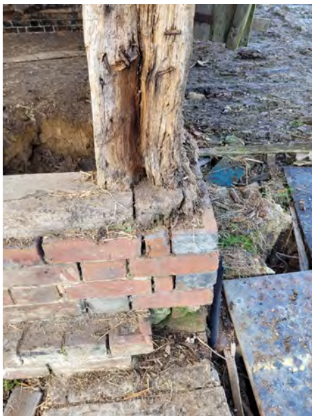
P89 Post base (Grid A9)
