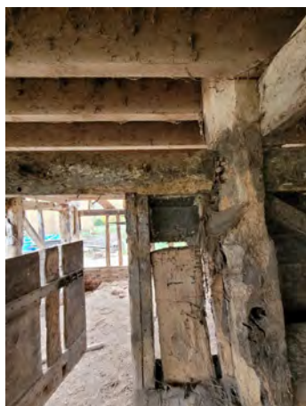
P79 Mid-rail (Grid B7)
