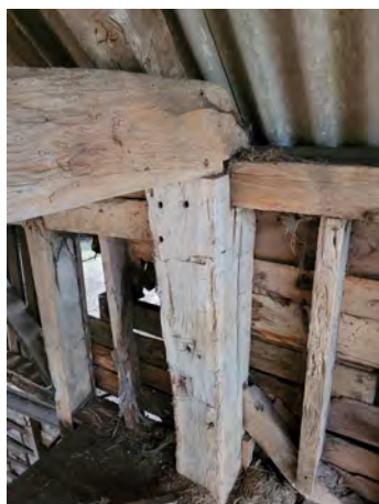
P33 Post to tie (Grid C3)
