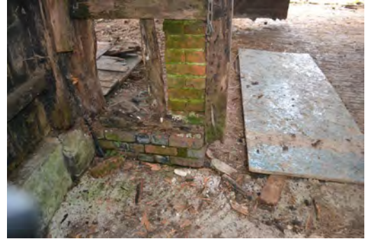
P42 Door post (Grid C4)
