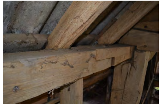
P53 Eaves splice (Grid 5C)
