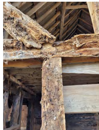
P98 Mid-rail brace (Grid C9)
