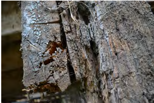
P19 Spine floor beam end (Grid B1)
