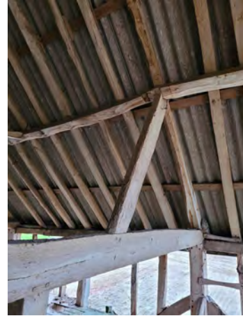
P70 Purlin strut (Grid A7)
