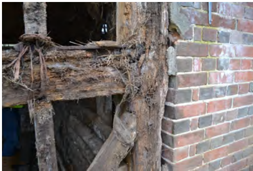
P15 Mid-rail to post (Grid C1)
