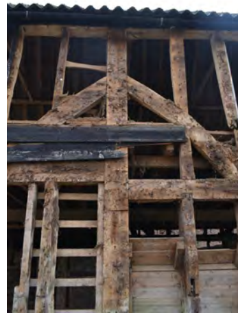
P65 Post to eaves (Grid A7)
