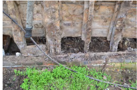
P20 Post base (Grid A2)
