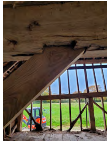
P32 Knee brace to tie (Grid C3)
