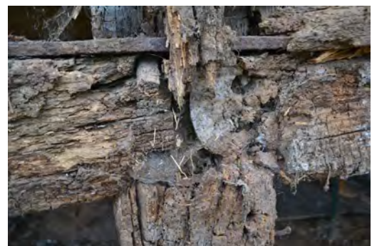
P12 Mid-rail tie (Grid B1)
