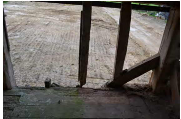
P104 Studs (Grid A6 to 7)
