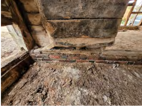
P81 Plate, cut brace (Grid A7)
