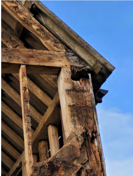
P91 Tie and brace (Grid A9)
