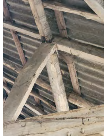
P30 Purlin strut (Grid A3)
