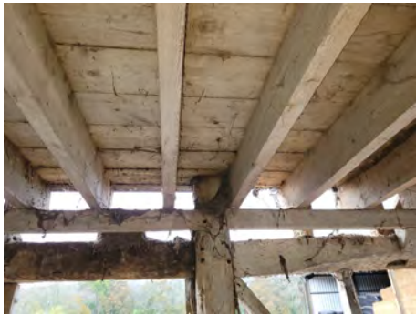
P83 Floor support (Grid A8)
