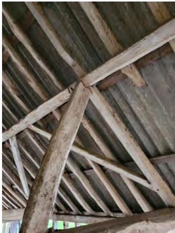
P48 Purlin strut (Grid A5)
