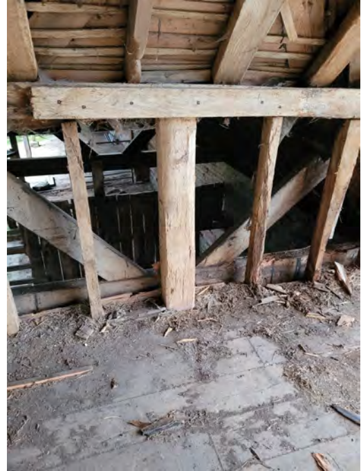
P26 Eaves splice (Grid C2)
