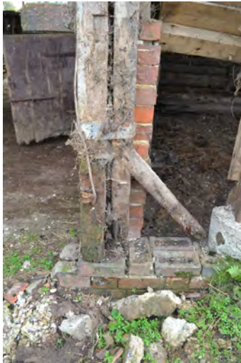
P37 Post base (Grid A4)
