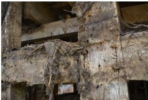
P21 Mid-rail (Grid A2)
