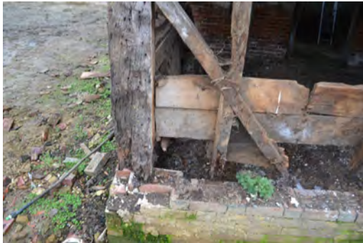
P7 Post and stud (Grid A1)
