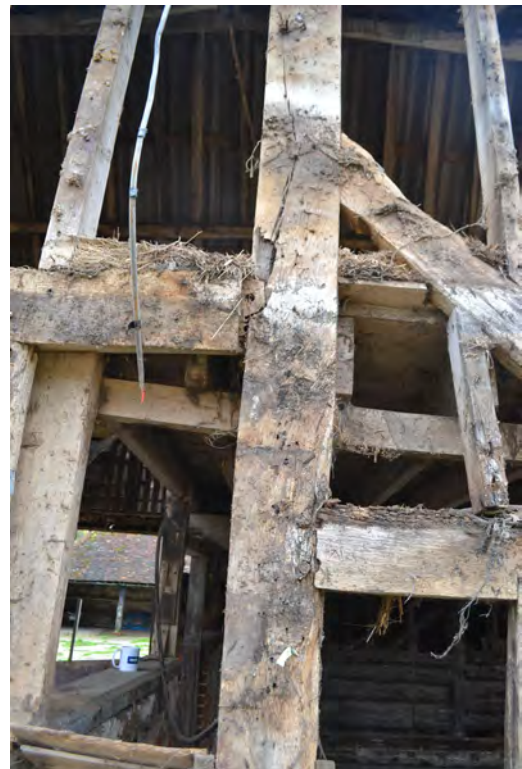
P28 Mid-rail (Grid A3)
