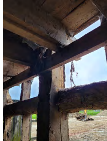
P59 Floor support (Grid A6)
