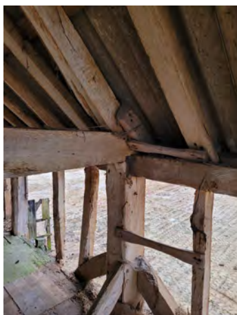
P68 Post bracing (Grid A7)
