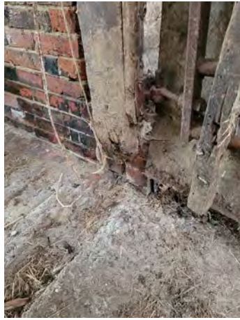
P52 Door post (Grid C5)
