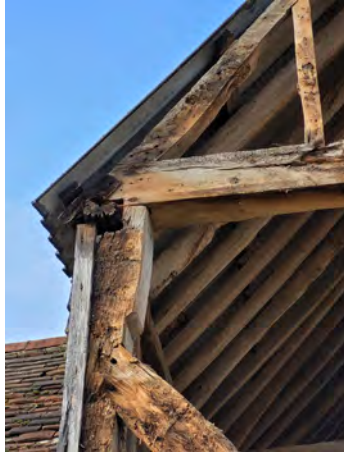
P101 Tie and brace (Grid C9)
