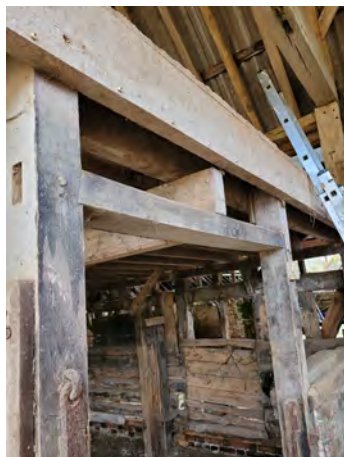
P54 Floor support (Grid B5)
