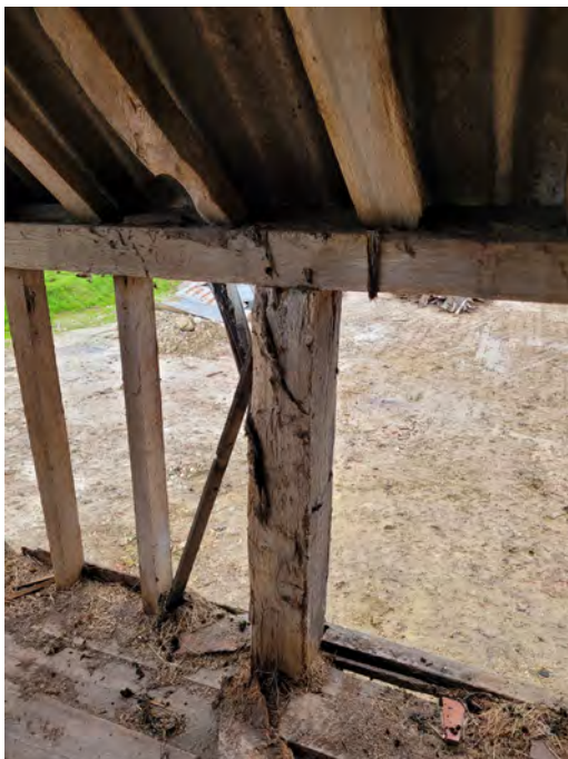
P23 Post to eaves beam (Grid A2)
