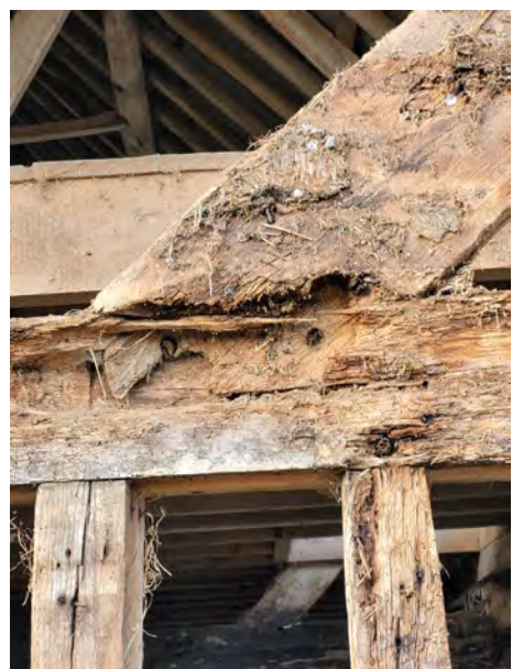
P94 Mid-rail brace (Grid A9)
