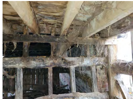
P18 Corner post to mid-rail (Grid C1)
