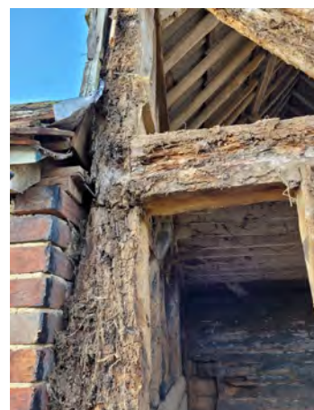
P100 Mid-rail (Grid C9)
