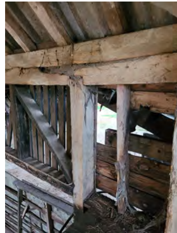
P43 Door post to eaves (Grid C4)
