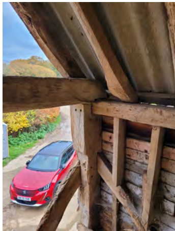
P103 Tie and eaves (Grid C9)
