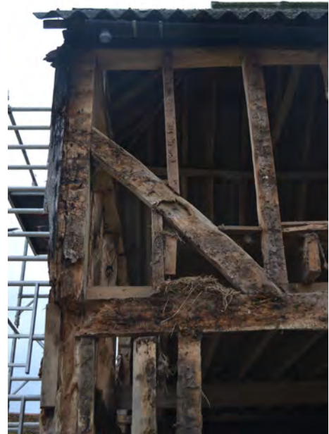
P88 Mid-rail (Grid A9)
