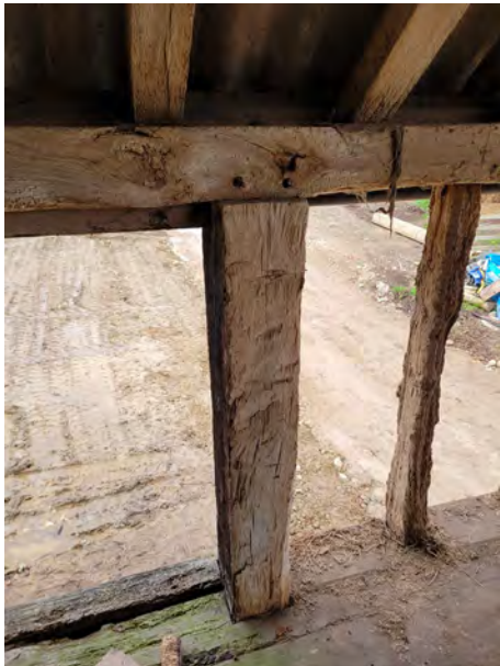
P85 Eaves beam (Grid A8)
