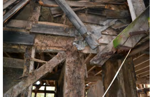
P76 Mid-rail and brace (Grid C7)
