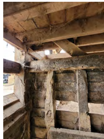
P67 Floor support (Grid A7)
