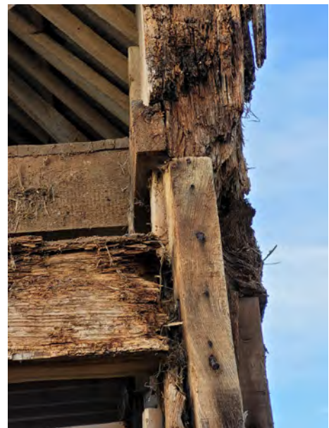
P90 Mid-rail (Grid A9)
