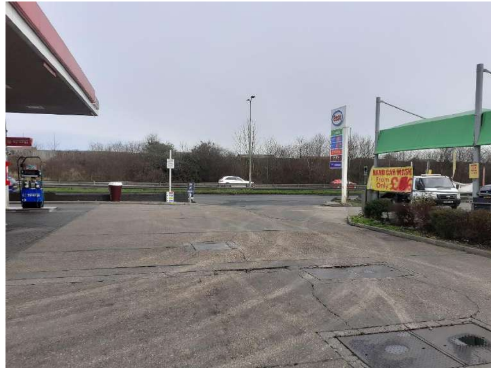
Photo 2: View of current UST farm looking north.
