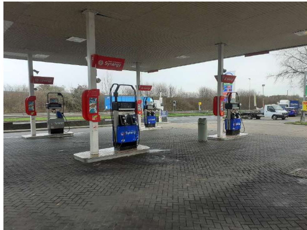
Photo 5: View of forecourt looking northeast.
