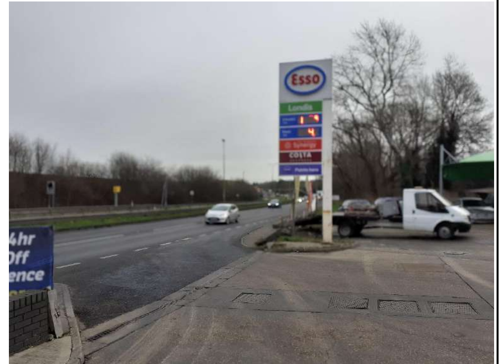
Photo 3: View of site egress and forecourt interceptor, in the northeast of site.
