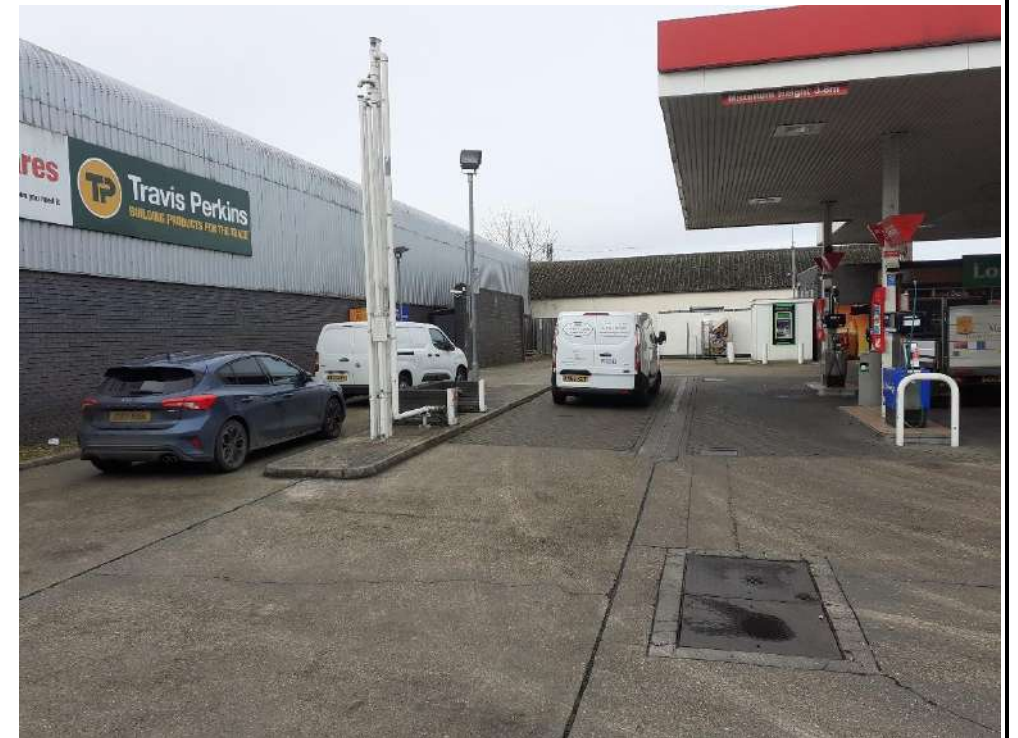
Photo 6: View of off-set fill points and tank vents, looking west.
