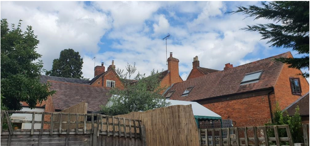
Context Photograph 6: The Royal Oak south (rear) elevation with modern extensions views from the driveway.
