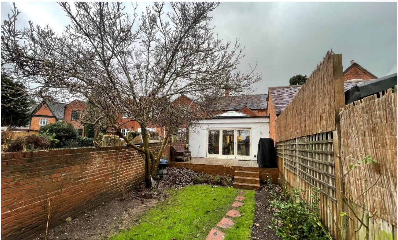
Context Photograph 2: South (rear) elevation and garden with modern flat roof kitchen extension c.2015.
