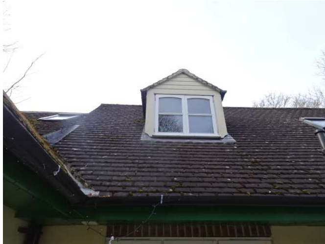
Roof area that will be affected by the development
