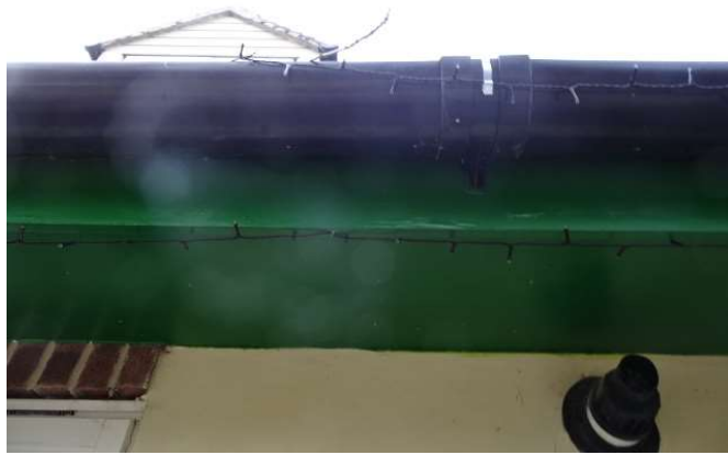
Wall top - sealed
