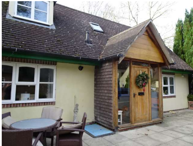
Front elevation showing existing porch
