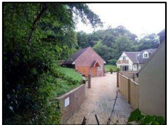
View of application site from drive / public footpath approaching from north
