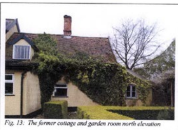
Fig. 13: The former cottage and garden room north elevation
