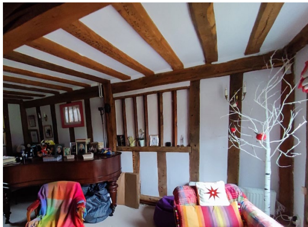
Existing blocked 6-light diamond-mullioned window in Snug to be re-instated.
