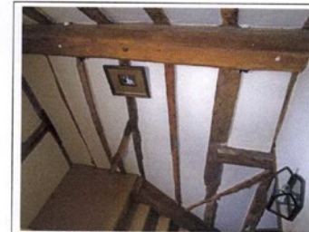
Fig. 23: Mid C18 framing in room F9, with two C17 studs to the right
