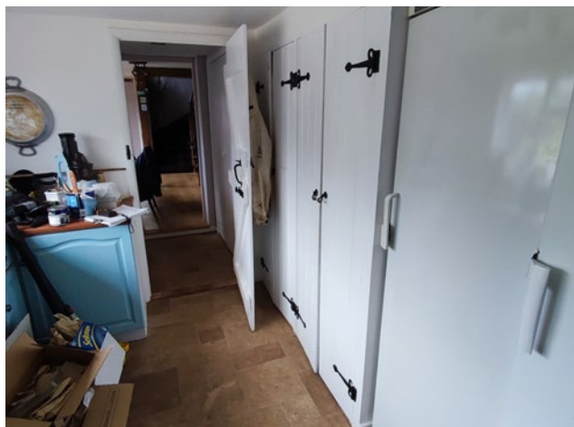
Modern stud walls to be removed to create proposed Garden Room.
