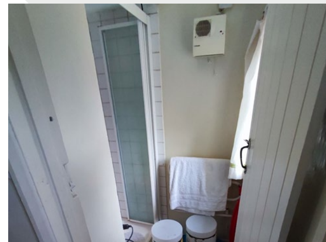
Existing Shower Room to be demolished.
