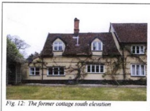
Fig. 12: The former cottage south elevation
