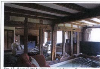
Fig. 17: Room G10A looking east to skeleton wall
