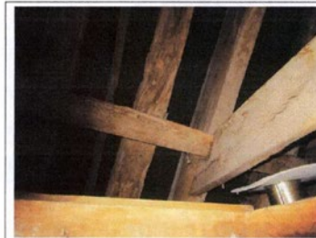
Fig. 22: Mid C18 roof detail
