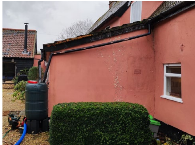
Partial demolition of lean-to to allow for proposed extension.
