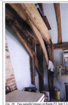
Fig. 20: Two parallel trusses in Room F3, late C15 and early C17
