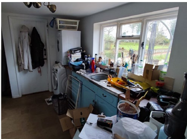
Utility to be relocated. Existing window to be removed and opening extended to provide glazed french doors and fixed glazed screens.
