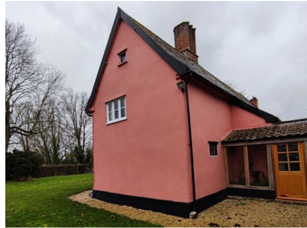
Infilled window to ground floor to be re-instated.
