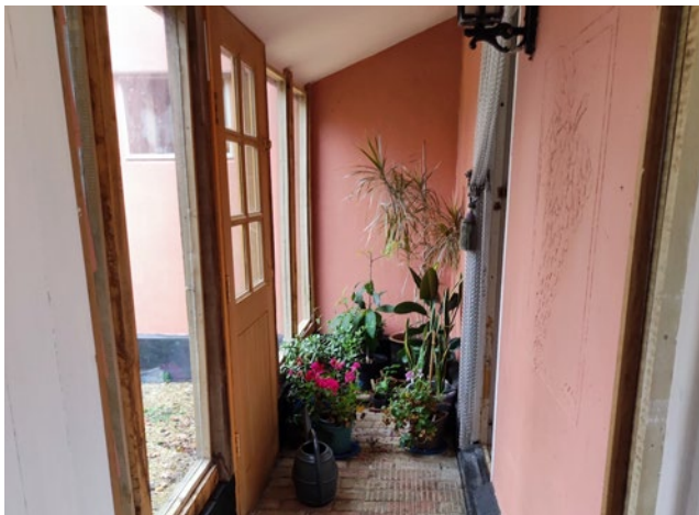
Retrospective: Infill glazed link creating lobby.
