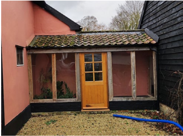
Retrospective: Glazed infill lobby created.
