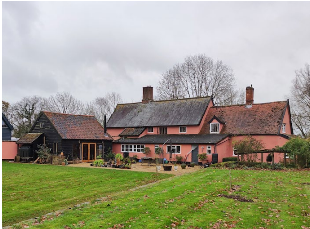
Later lean-to extension to be altered and extended. Retrospective: Reinstatement of historic first floor window.
