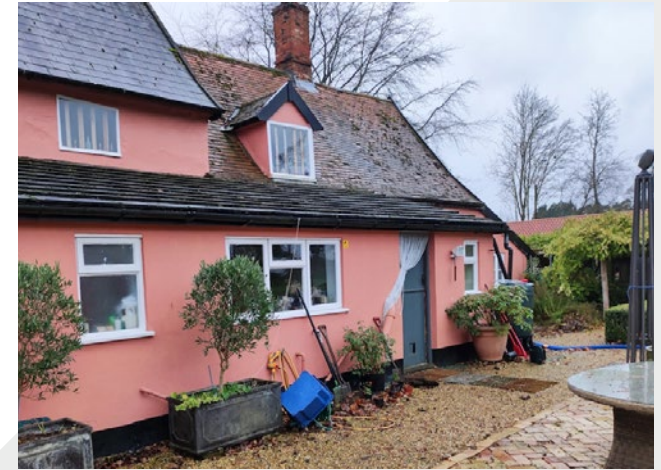
Utility window and door to be removed and replaced with glazed french doors and fixed glazed screens. Concrete roof tiles to be removed and replaced with natural slate.
