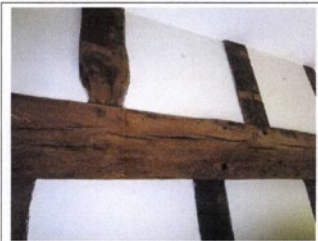
Fig. 21: Carpenter's marks on east truss in room F6
