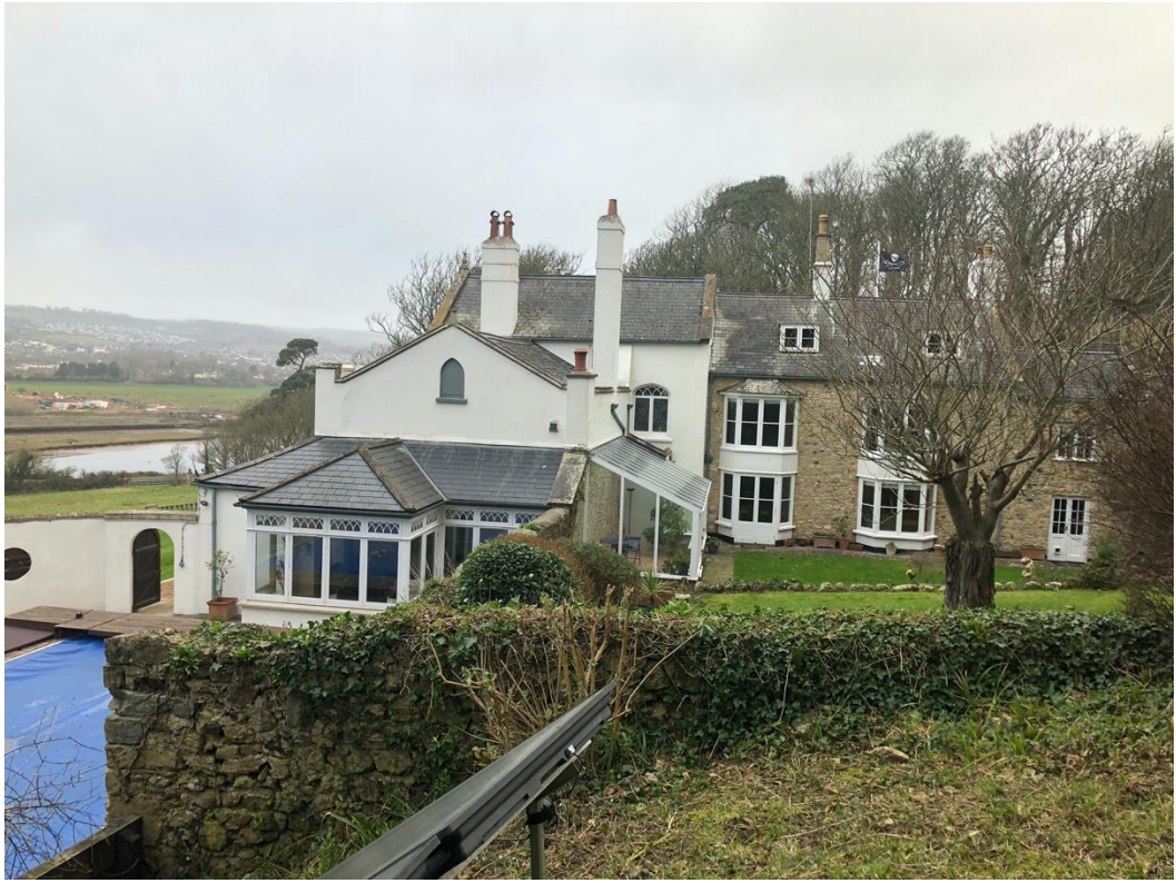
Figure 2: South East Elevation
