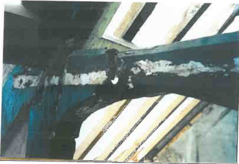
Repair of fractured door head
