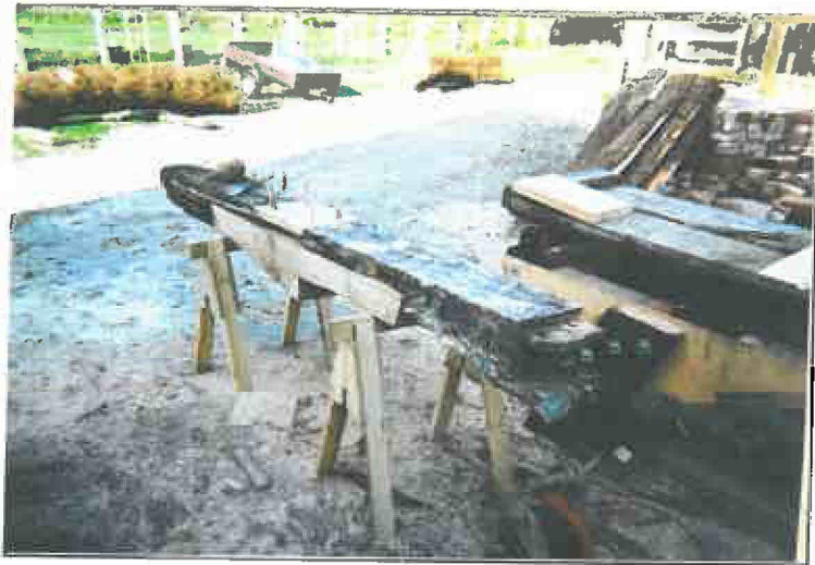
Ready to re-install
