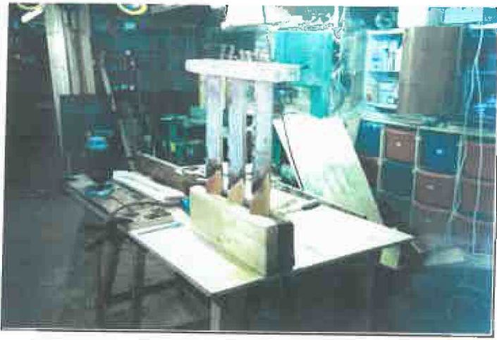
Repair of timber mullion window
