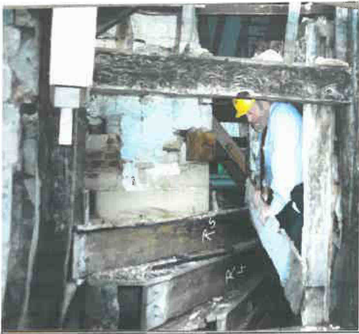
Carefully numbered for dismantling and assessment
