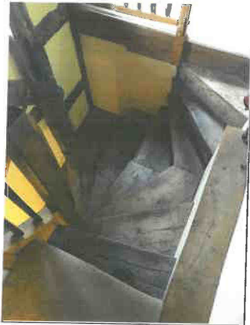
Descending Appendix V Yew Tree Farmhouse
