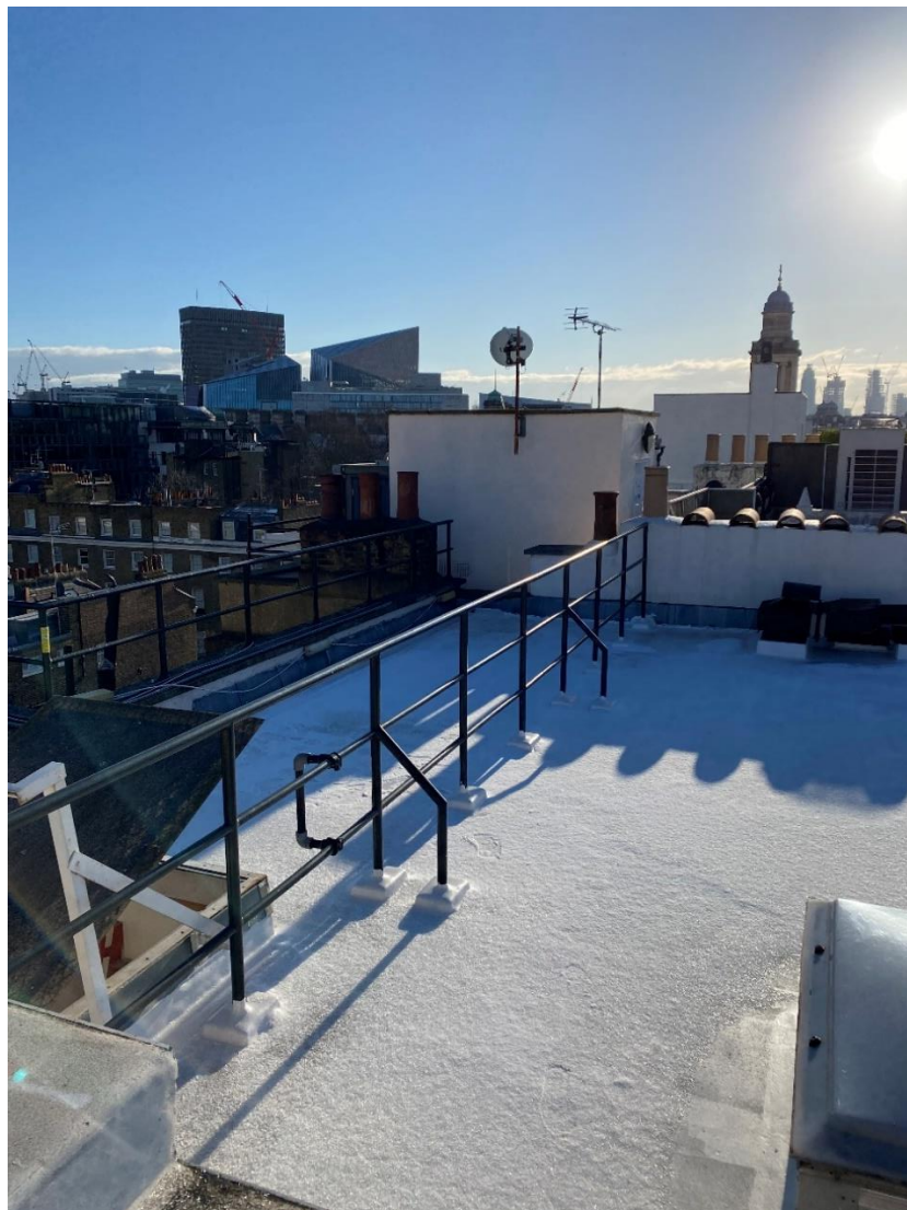
Photo 1 – Roof of 7-8 Upper Belgrave Street
