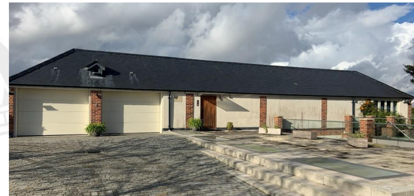
South east elevation of converted outbuildings at Windmill Farm
