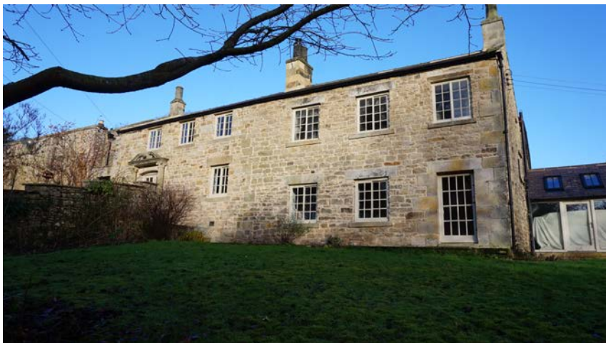
Plate 3 - southern elevation of main house - looking northwest from the garden
