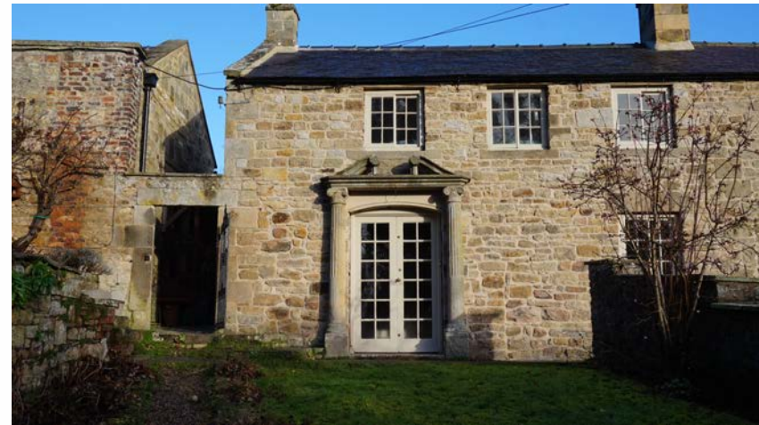
Plate 10 - door surround with fluted columns and broken scroll pediment
