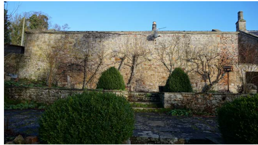
Plate 2 - area of terracing and location of former glasshouse - looking north
