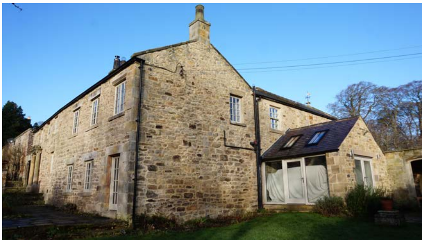
Plate 11 - eastern elevation of Appletrees and garden room built in 2014 - looking northwest
