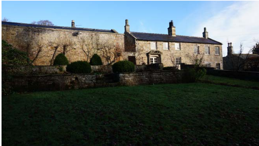
Plate 9 - southern elevation of Appletrees viewed from the south garden
