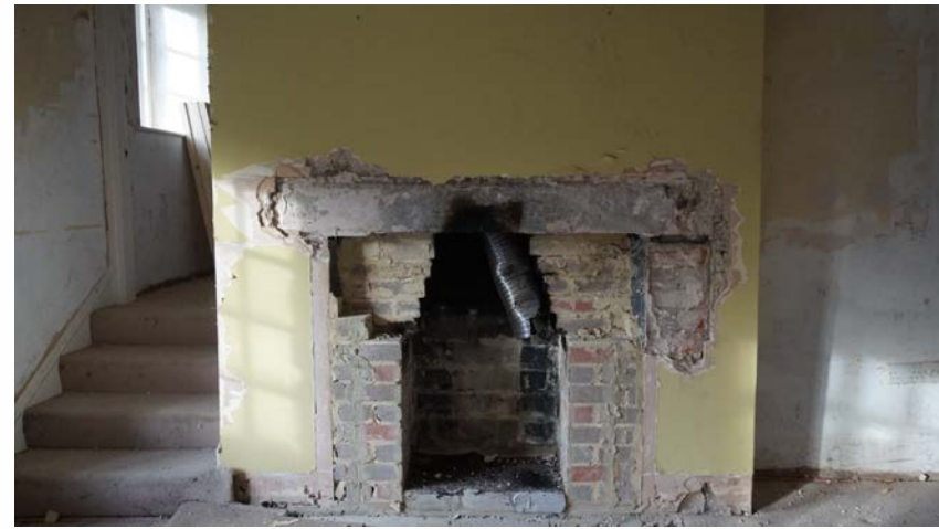
Plate 22 - modern brickwork to accommodate log burning stove
